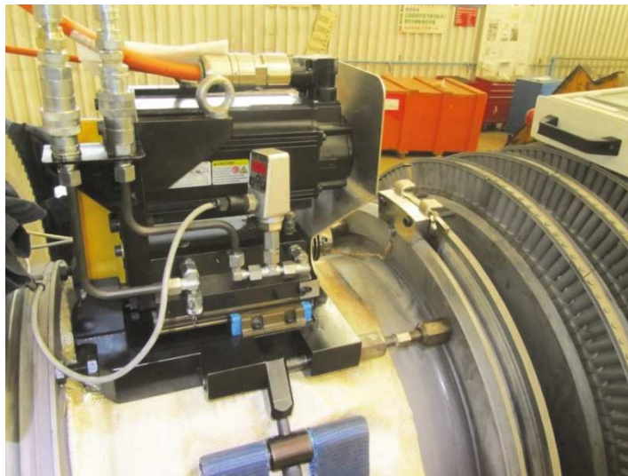
Figure 1. Illustration of the bespoke FTHP platform in position on a stream turbine rotor. It uses the registered WeldCore® process and is capable of extracting an annular metallurgical sample through the thickness of the blade attachment t-slot wall, repairing and re-drilling the hole in a single sequence of operations.
