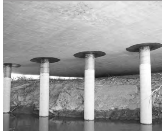
Figure 4. Highway structure with silicone paint surface modification.
