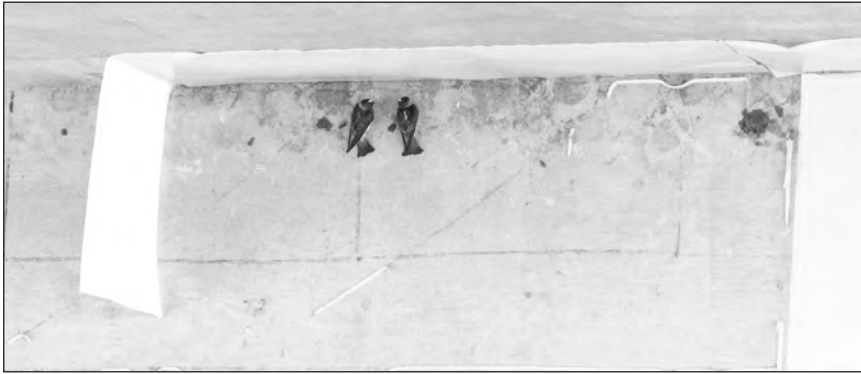
Figure 10. PTFE sheets detaching from the concrete bridge surface and cliff swallows building nests.
