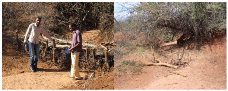
A pair of photos showing (left) an intact sieve structure and (right) the same structure destroyed by flooding in the heavy spring rains. All the branch packing, the large ballast logs, and most of the upright stubs have been washed away in the right photograph. (Photo credits: (left) Brien E. Norton and (right) Bedasa Eba).
