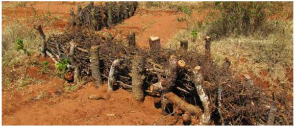
A pair of sieve structures at the confluence of 2 secondary gullies in the Dikale enclosure. The basic design consists of two rows of tree stubs sunk into the gully floor and packed with acacia branches. Some excavation has occurred in sand at the base of the sieve near the camera due to animal activity. (Photo credit: Brien E. Norton).
