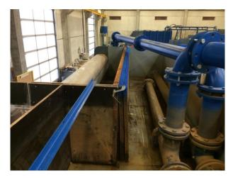
Figure 3. Upstream view of the facility: reservoir, water supply pipes and baffle wall upstream of the right side crest.
