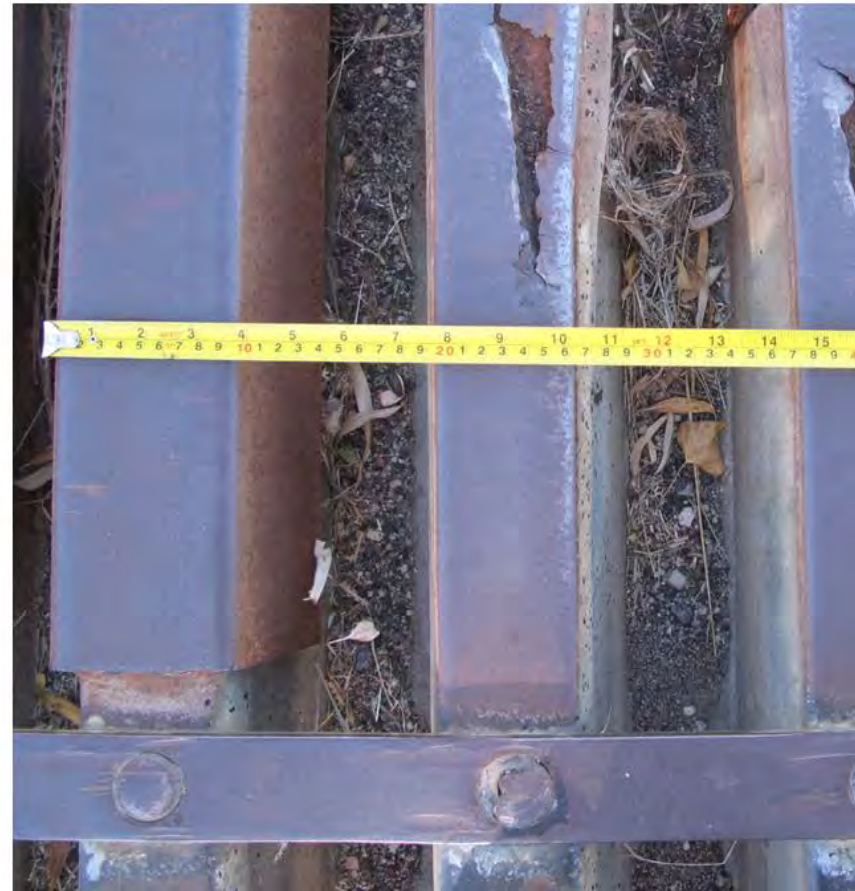
Figure 2. Cattle guard (1.9-m \times 9.7-m) not constructed over excavation (A) and close view of cattle guard rails (B) on an access road to Interstate 15, near Summit, Utah, USA.
