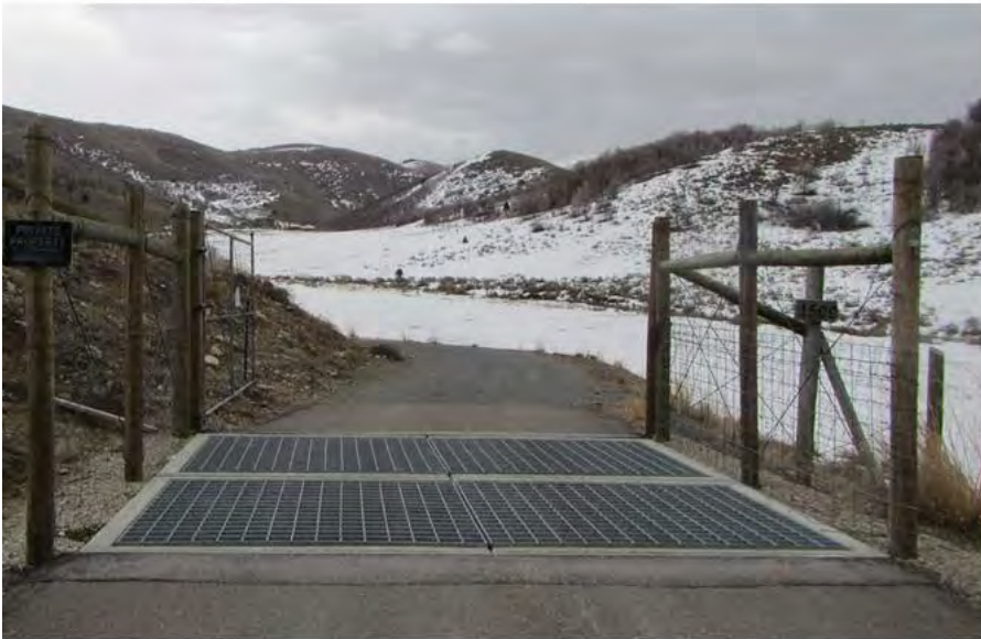
Figure 5. Wildlife guard (4.9-m × 4.9-m) suspended over excavation (A) and close view of steel grating (B) on an access road to U.S. Highway 91, near Mantua, Utah, USA.
