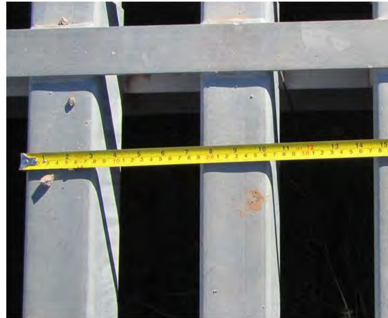
Figure 3. Standard cattle guard (2.1-m × 11-m) suspended over excavation (A) and close view of cattle guard rails (B) on an access road to Interstate 15, near Pintura, Utah, USA.
