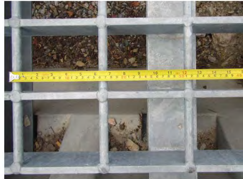
Figure 5. Wildlife guard (4.9-m × 4.9-m) suspended over excavation (A) and close view of steel grating (B) on an access road to U.S. Highway 91, near Mantua, Utah, USA.
