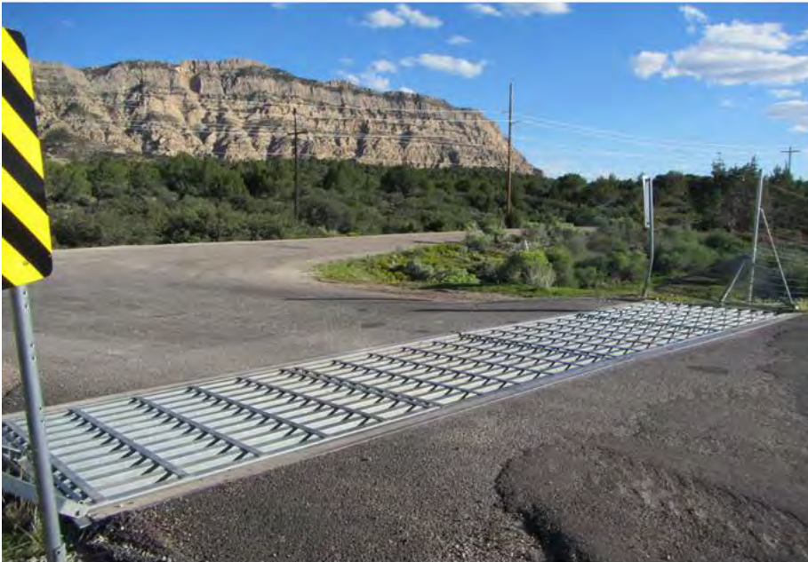
Figure 3. Standard cattle guard (2.1-m × 11-m) suspended over excavation (A) and close view of cattle guard rails (B) on an access road to Interstate 15, near Pintura, Utah, USA.
