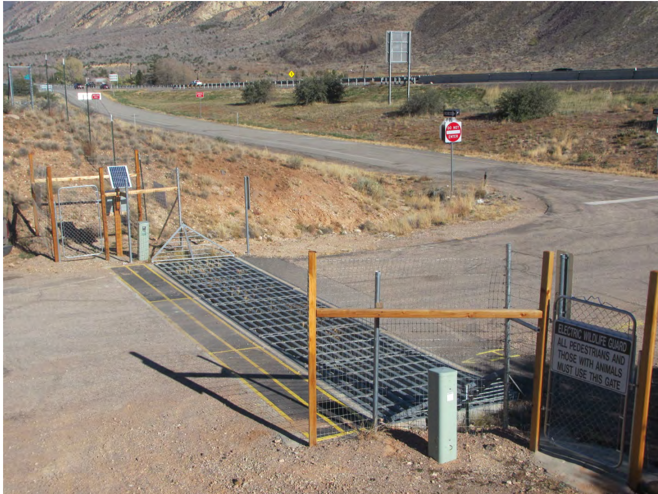
Figure 13. Cattle guard (2.1-m \times 11-m) augmented with electrified pavement (0.91-m \times 11-m) on access road to Interstate 15 (background), near Pintura, Utah, USA.
