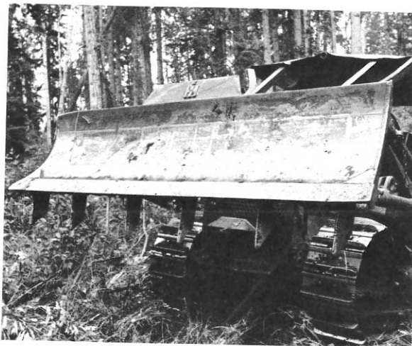
Figure 11. Crawler-type tractor with a 6-toothed bulldozer blade, 9 feet wide.
