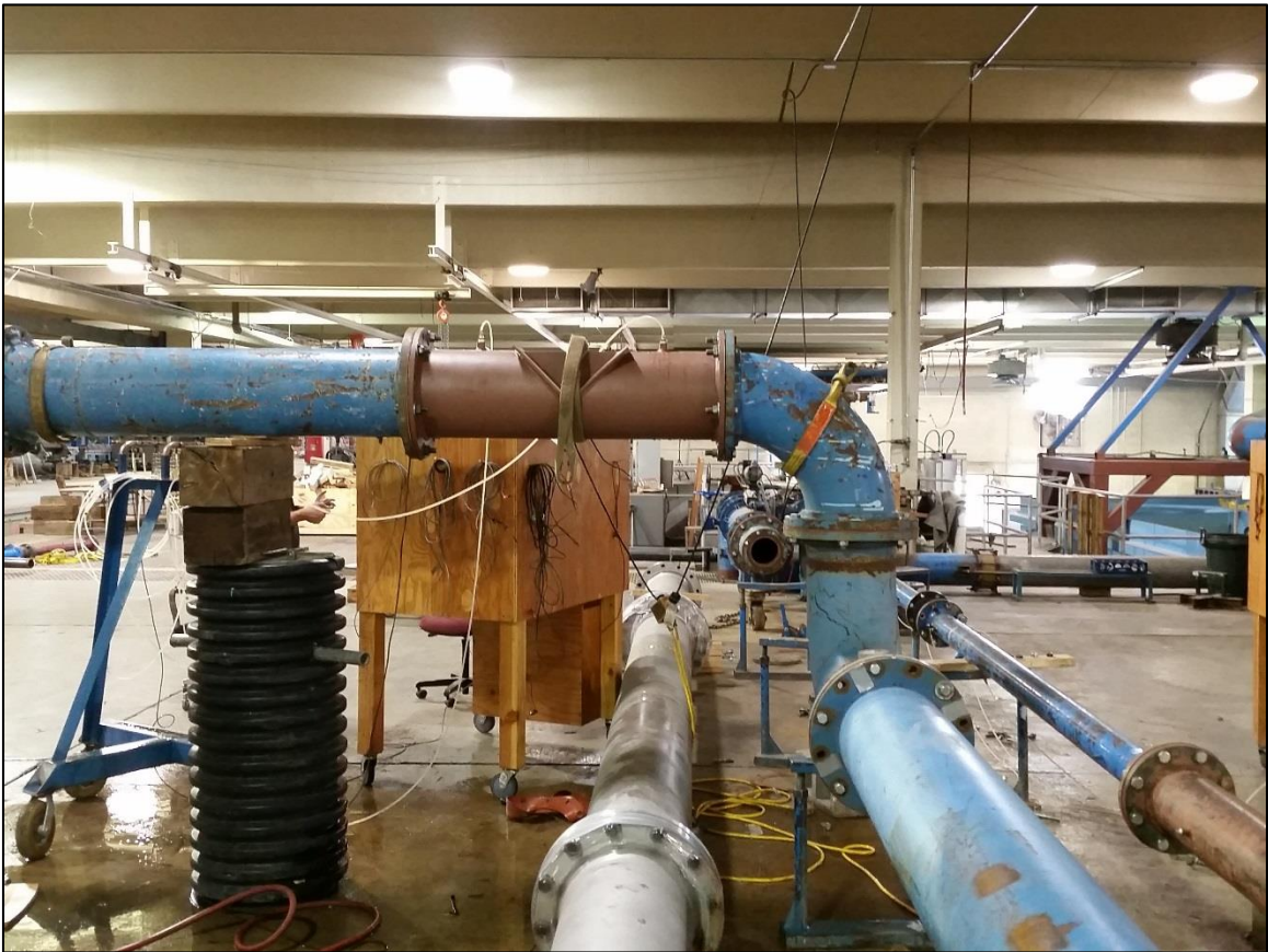
Figure 4: Wedge Flowmeter Close Coupled to DEOP in the Vertical Position
