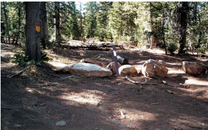
Rocks and logs have been placed to block access to this closed road.
