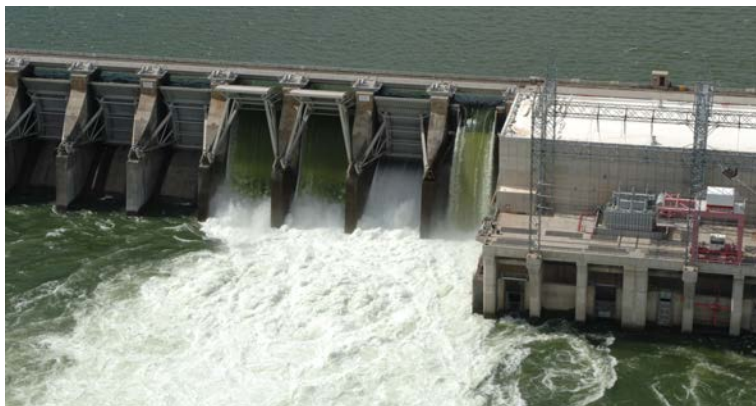
Figure 5. Topspill in bays 19, 20, and 22 and bottom spill in bay 21 as tested in 2008.
