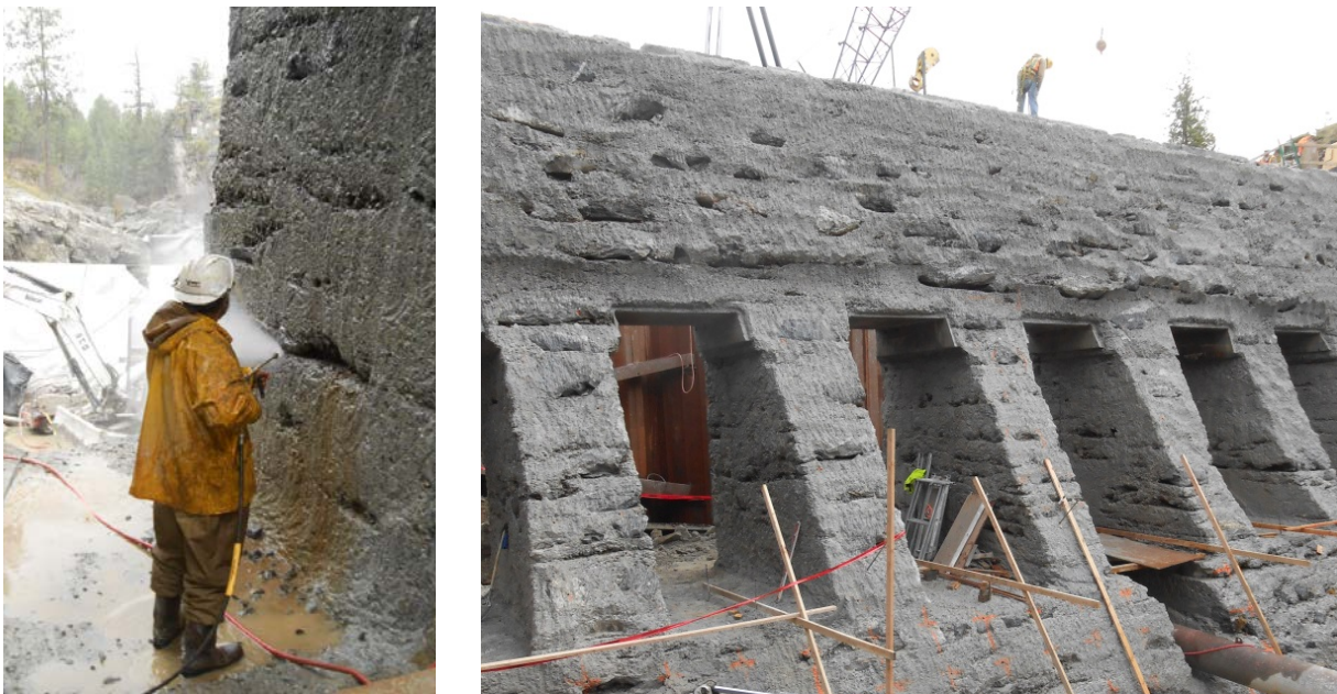
Figure 5. Concrete Demolition and Surface Preparation
