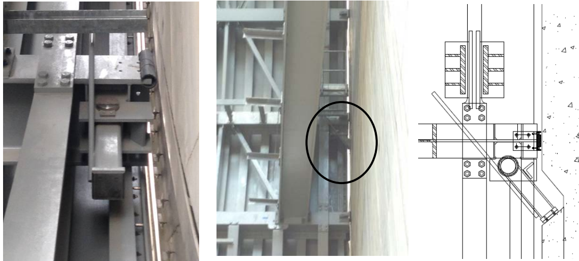
Figure 8. Dogging Devices (Circled) - Engaged and Disengaged
