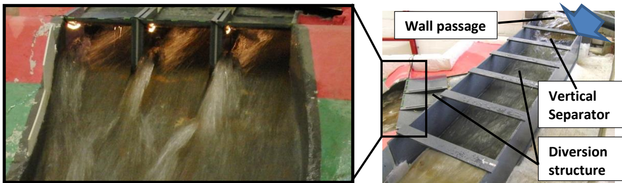
Figure 7. View into the three channels of the lower diversion structure (left) and at the upper diversion structure (right) in the optimized state in the hydraulic model, load case HQ_{1,000}
