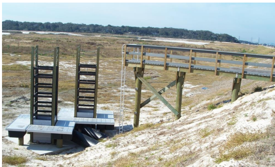
Figure 4. Set of 4.9 m (16 ft) tall 1.2X1.2 m (4x4 ft) Box Riser Weirs with floating dock access, Buck Island, Jacksonville, Florida. (Maglio et al. 2014).
