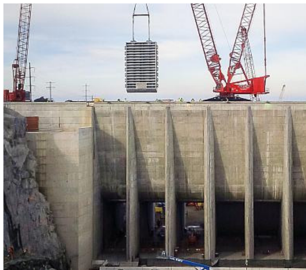
Figure 15. Folsom Spillway Bulkhead, USA (U.S. Bureau of Reclamation/USACE [Frank 2015])
