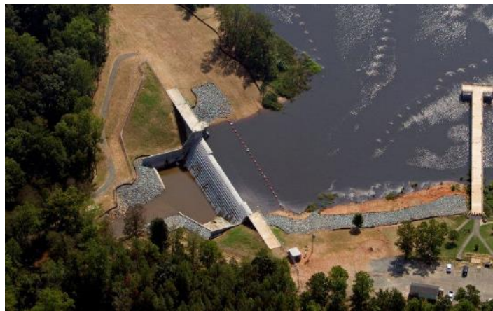
Figure 4. Overview of Salem Lake Dam
