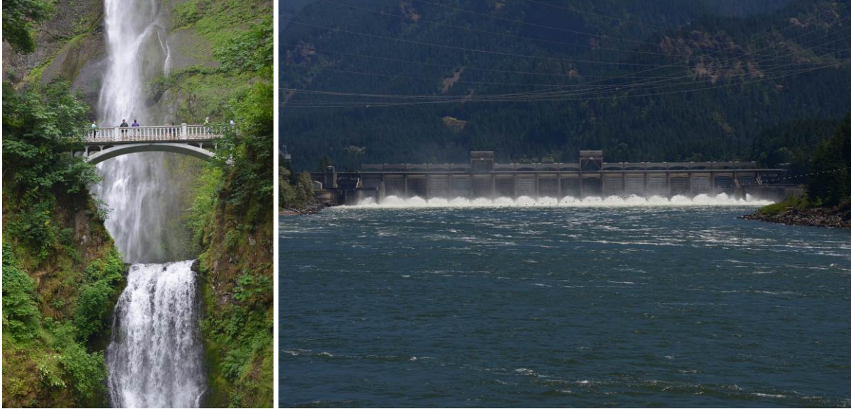
Figure 3. Multnomah Falls and Bonneville Dam Spillway (photos courtesy Brian Crookston)
