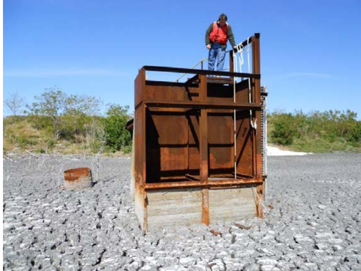
Figure 1. Box riser weir crevice corrosion at water-air interface after one use cycle.
