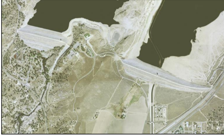
Figure 1. Isabella Main Dam and Auxillary Dam
