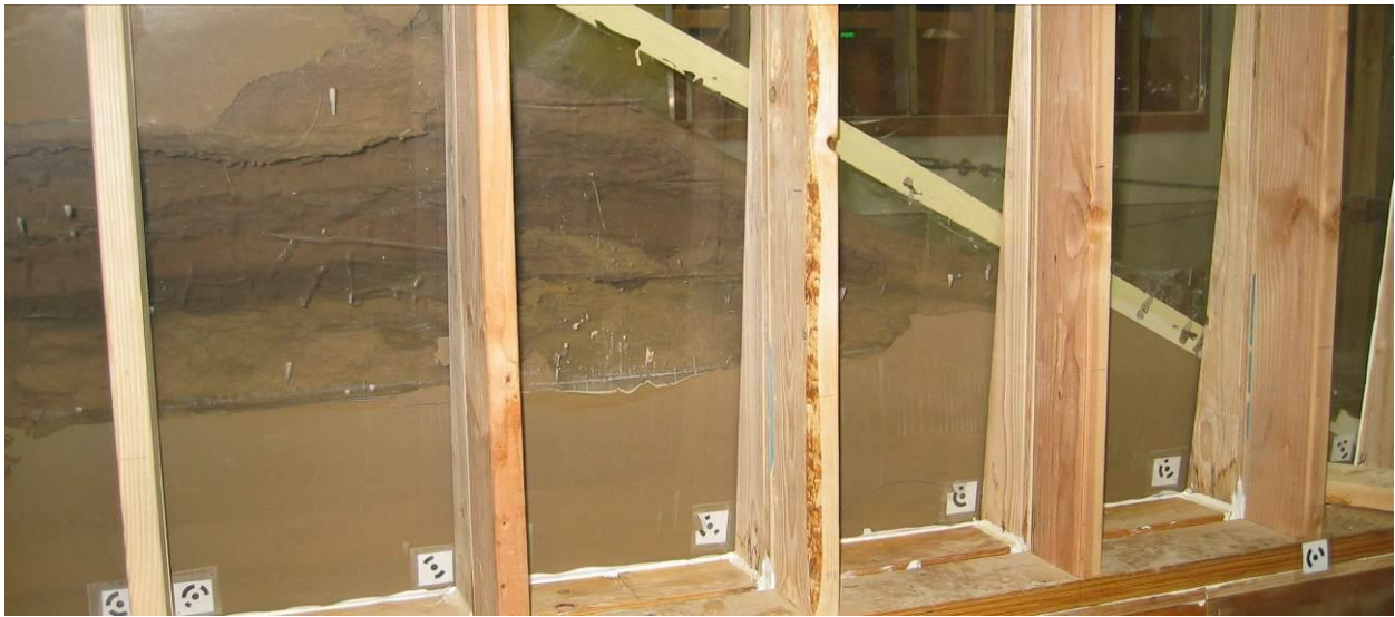
Figure 7. Post-test photo illustrating significant widening of the erosion channel, especially near its base.
