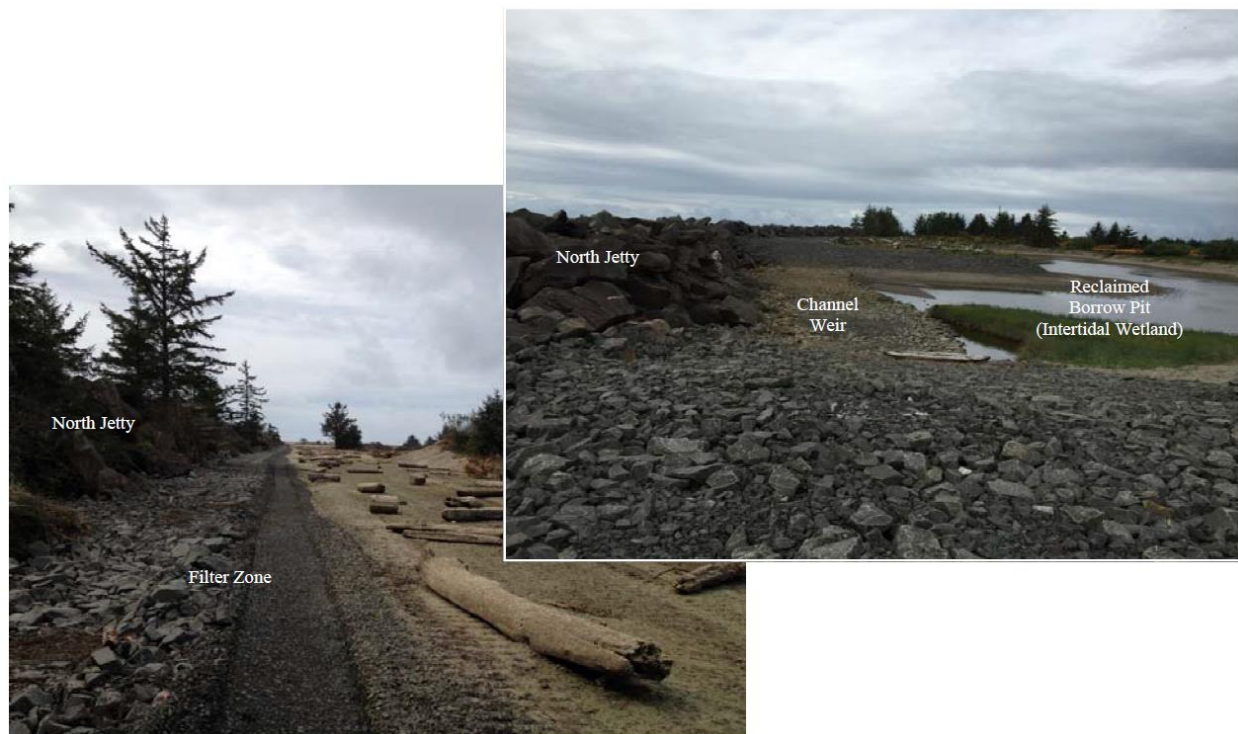
Figure 9. Looking west toward lagoon fill filter zone (left), and channel weir and reclaimed borrow pit (right).
