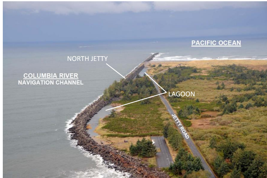
Figure 1. North Jetty lagoon aerial photograph looking southwest
