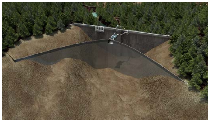
Figure 8: 731 M wide, 91 M deep guide net built of Dyneema®
