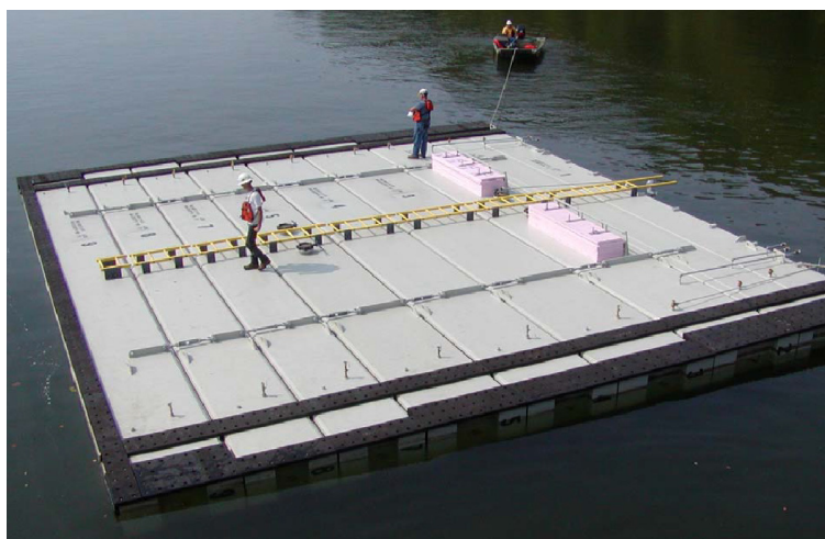
Figure 8. Hinged Floating Bulkhead, USA (Tennessee Valley Authority)
