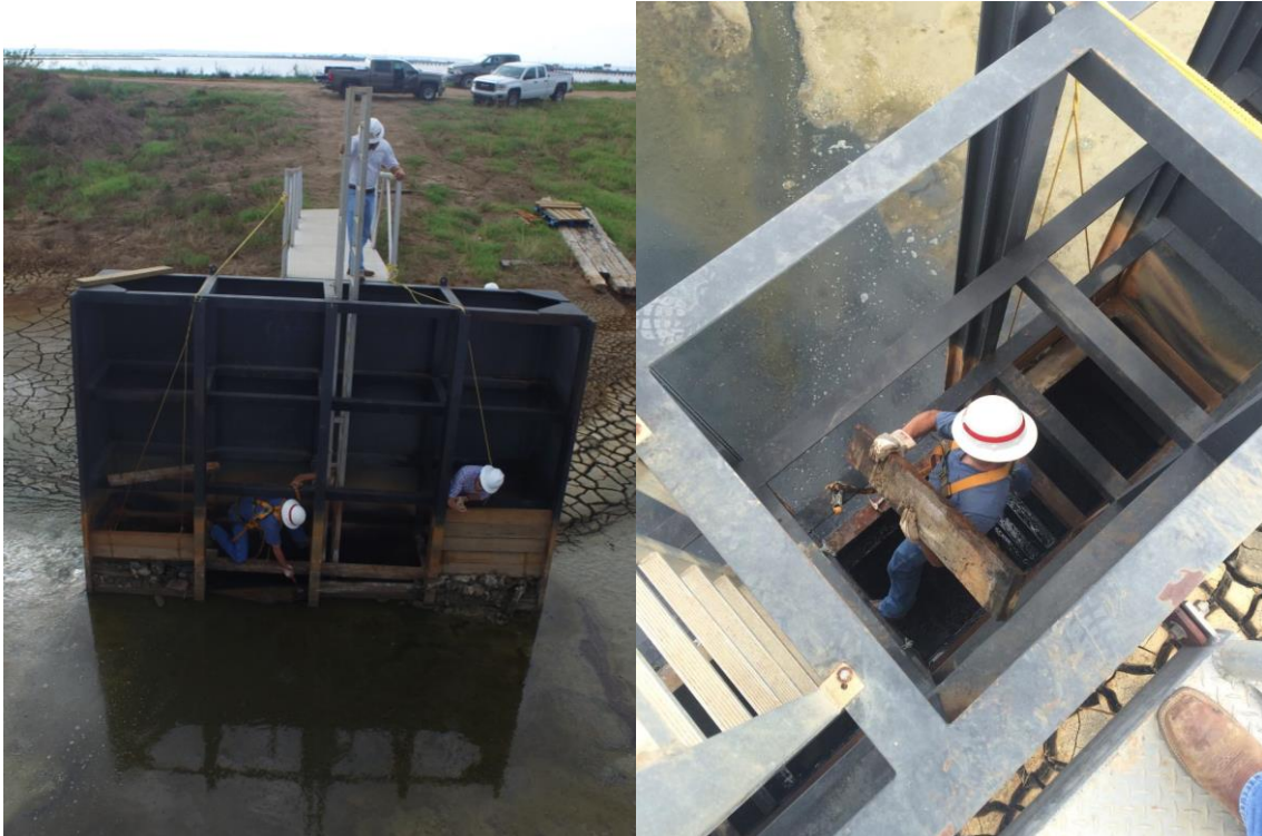
Figure 3. Traditional USACE fluid control operation (removing timber weir boards) with harnesses within confined disposal area (front view - left) and (plan view - right).
