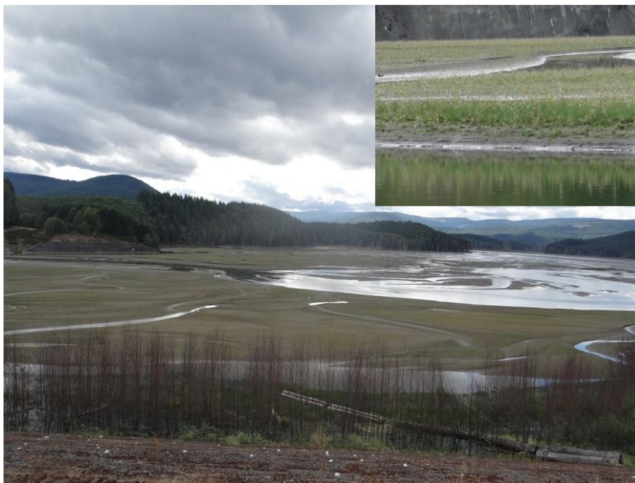
Figure 5. Conditions upstream of SRS spillway raise in summer 2013
