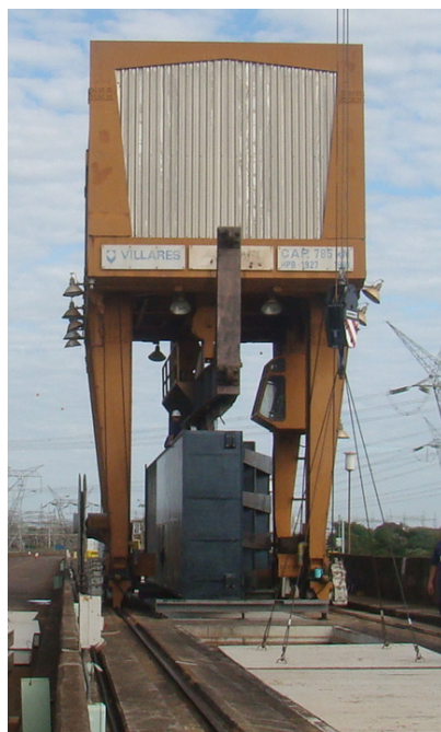
Figure 1. Stoplog Install, Itaipu Dam, Brazil/Paraguay (Itaipu Binacional)
