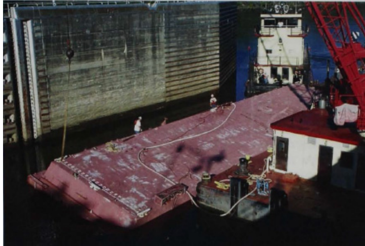
Figure 7. Floating Caisson Being Ballasted, USA (USACE Nashville District, ERDC/GSL TR-10-44)
