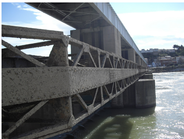
Figure 12. Flix Dam Stoplogs, Spain (Endesa)
