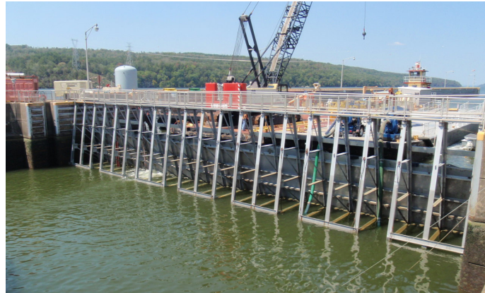
Figure 2. Poirée Needle Dam, Dardanelle Lock and Dam, USA (USACE Little Rock District)
