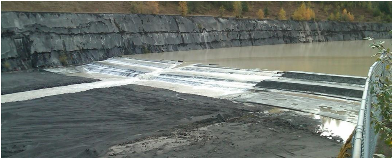
Figure 9. Completed spillway raise, 17 October 2012
