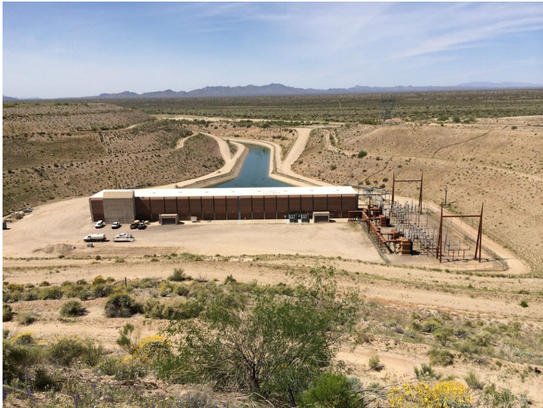
Figure 5. Hassayampa Pumping Plant
