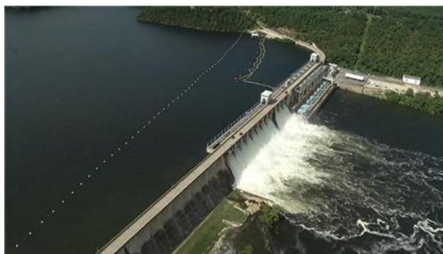
Figure 10. Gated spillway at Bagnella Dam, Osage River, Camden
