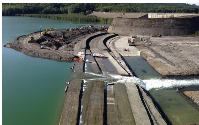
Figure 8. SRS spillway raise during construction
