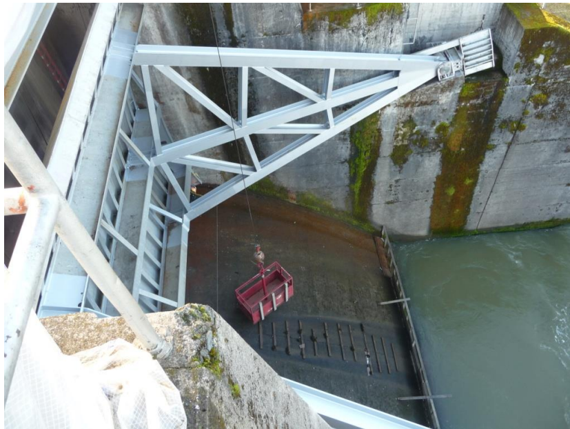
Figure 3. New End Frame at Dexter Dam Spillway Gates, Lowell, Oregon.
