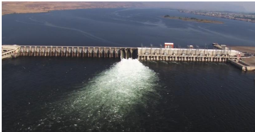
Figure 8. Photograph of the final fish bypass in operation.
