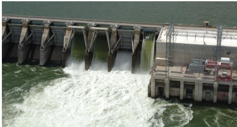
Figure 5. Topspill in bays 19, 20, and 22 and bottom spill in bay 21 as tested in 2008.
