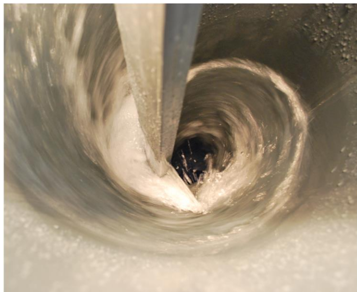
Figure 8. side view of the central air core at the inlet of the vertical drop shaft for scenario D
