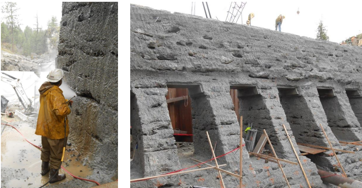
Figure 5. Concrete Demolition and Surface Preparation
