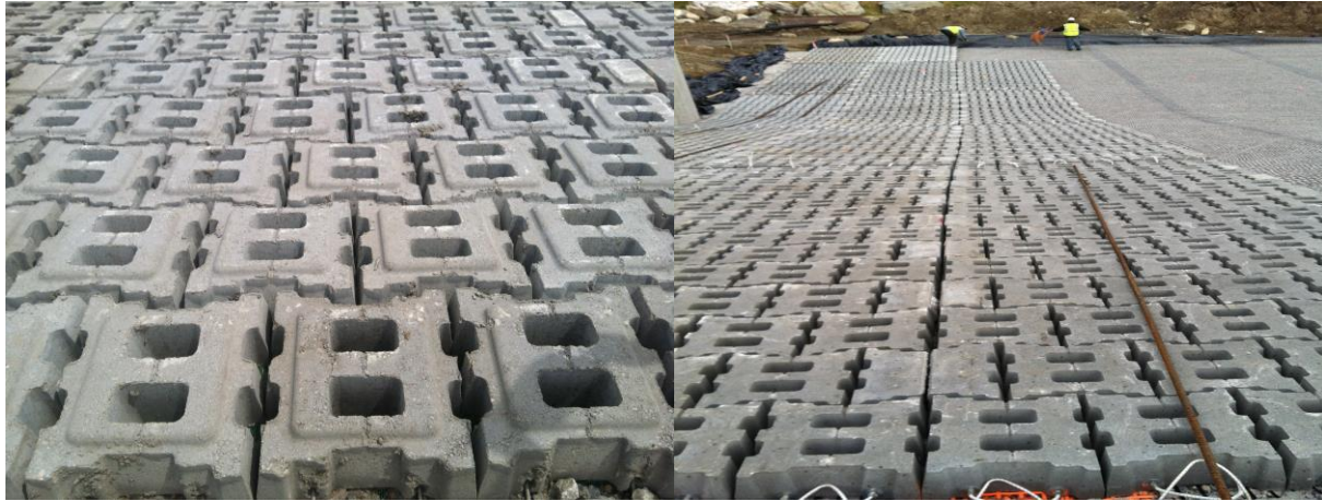
Figure 5. Interlocking Dome Top ACBs
