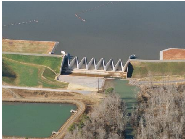
Figure 1. Overview of Lake Townsend Dam
