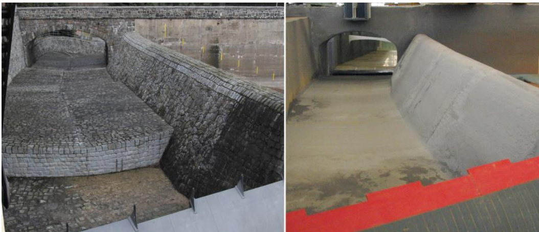
Figure 3. Spillway of the Malter Dam 2014 (left) (Source: LTV); Evened bottom slope in the hydraulic model (right)
