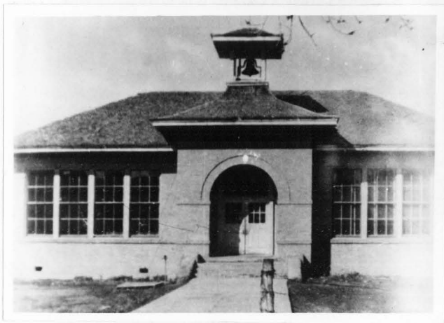
Fig. 14--Fayette Schoolhouse, completed in 1927.
