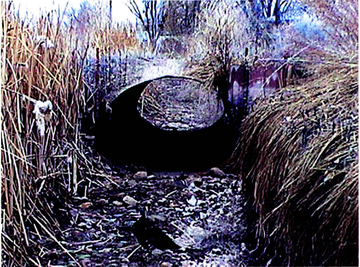
Figure A-D2 Green River Canal culvert crossing (no fine sediment deposition).
