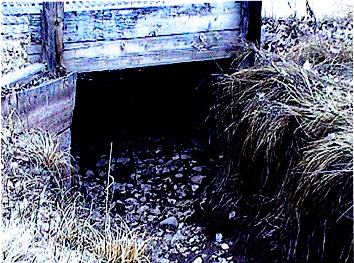
Figure A-D1 Green River Canal bridge crossing (no fine sediment deposition).
