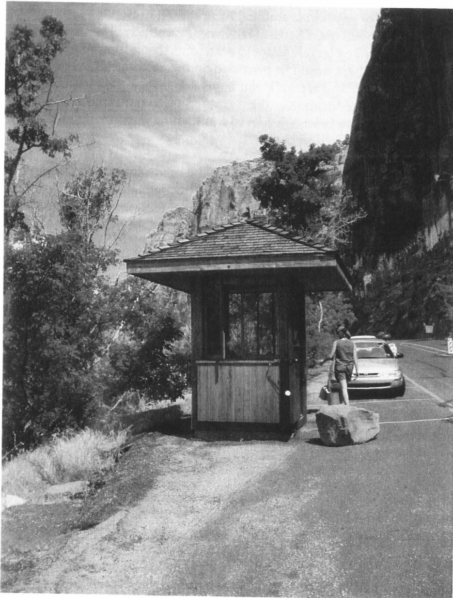
FIGURE 11. EXISTING RANGER KIOSK
