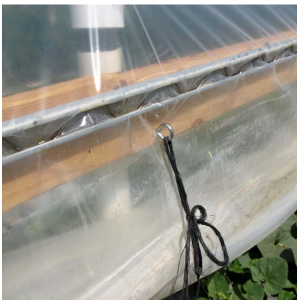
Figure 10. Wiggle wire holds the plastic in the track. Eye screws are used for both anchoring and ventilation.
