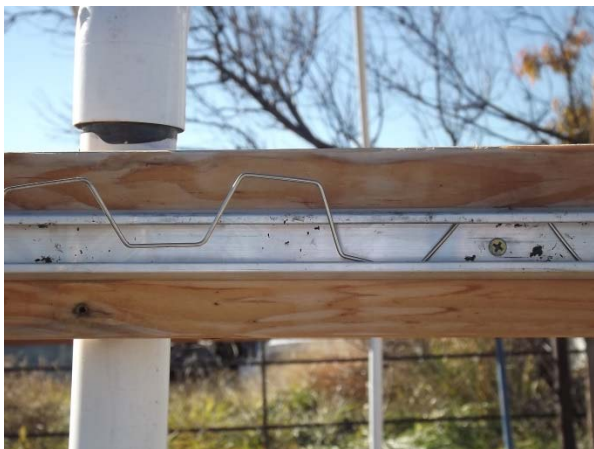
Figure 9. Wiggle wire and track fastened to the purlin.
