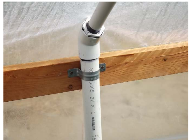
Figure 2. This joint assembly has been glued. Note the reducer in the 45° elbow so the arch pipe is 1 inch. The pipe clamp holds the purlin in place.
