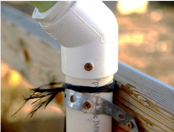
Figure 3. This joint assembly is stabilized with a grabber screw and can be disassembled if desired.
