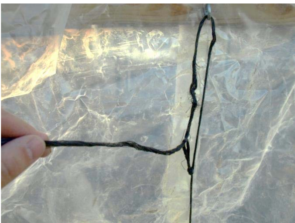
Figure 13. Run the cord through the eye screw and back through the loop.
