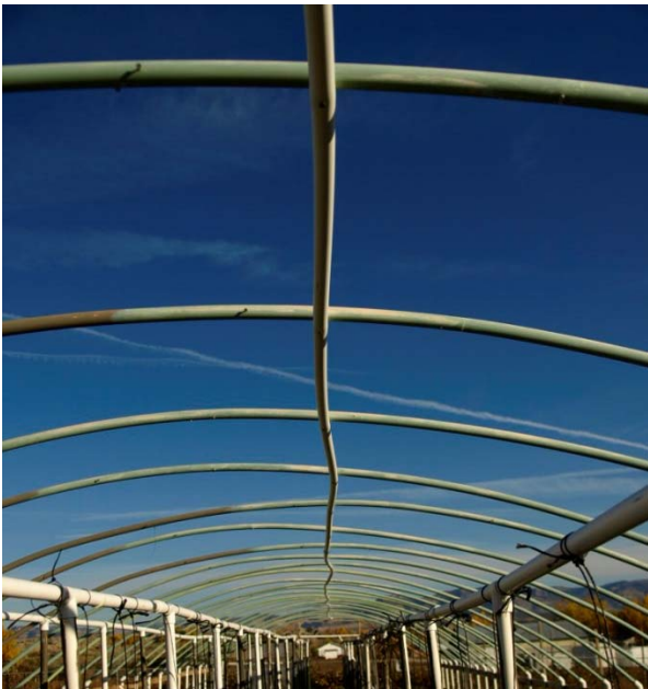
Figure 4. The ridge purlin will keep the roof ribs evenly spaced.
