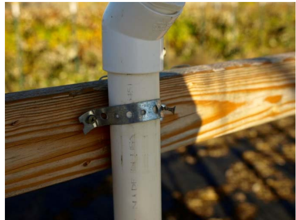
Figure 8. Plumber's strap can be used to hold the purlin to the sidewall. A screw will hold the purlin up until the covering is in place. Then the screw can be removed and the anchor ties can be used to keep the cover taut.
