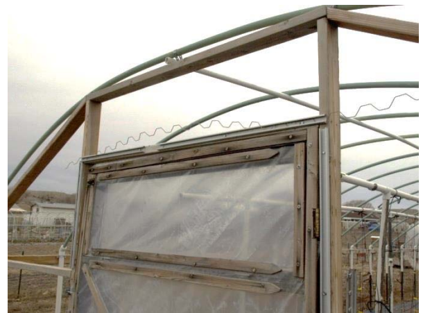
Figure 15. Wiggle wire track can be fastened to the door frame to aid in attaching the end wall plastic.
