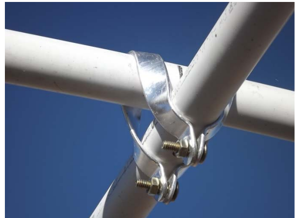
Figure 6. Aluminum cross connectors are designed to hold two pipes perpendicular to each other and can be adjusted to the right position before they are tightened. Measure outside diameter of pipe to ensure they fit over the ribs and purlins.
