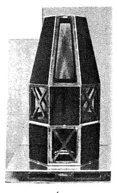
Figure 1 FORTÉ Bus Structure Shown with only a few solar panels installed.
