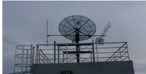
Figure 2 NTU Ground Station
