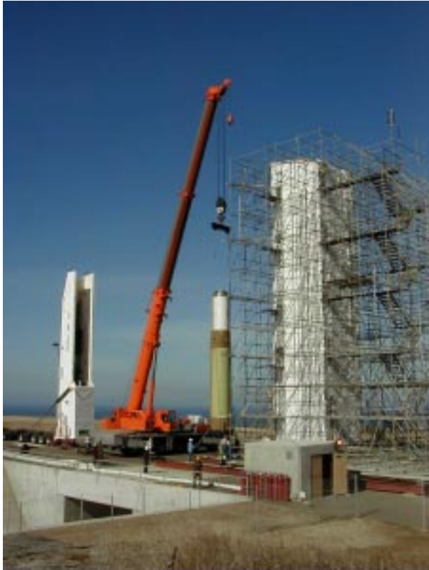
Figure 14 - Lower Stack Assembly Emplacement
