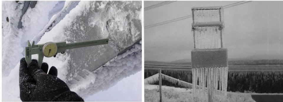
Figure 2-2: Atmospheric ice accretions on transmission line towers
