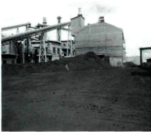
Figure 4.1 Coke pile in the outside yard
