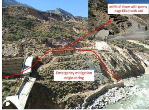
Fig. 15. Artificial slope (photograph taken 12 th December 2015).
