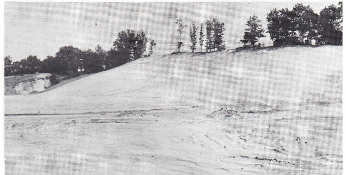
Shows bank shaped to a 3:1 and compacted ready for seeding.
