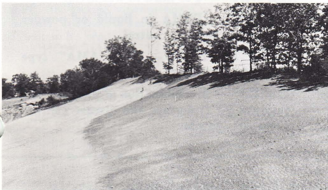
Dark area in right foreground shows area that has been limed, fertilized, seeded and mulched.
