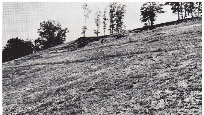
In September, two months after seeding, the area is stabilized and there is little or no sand blow.
