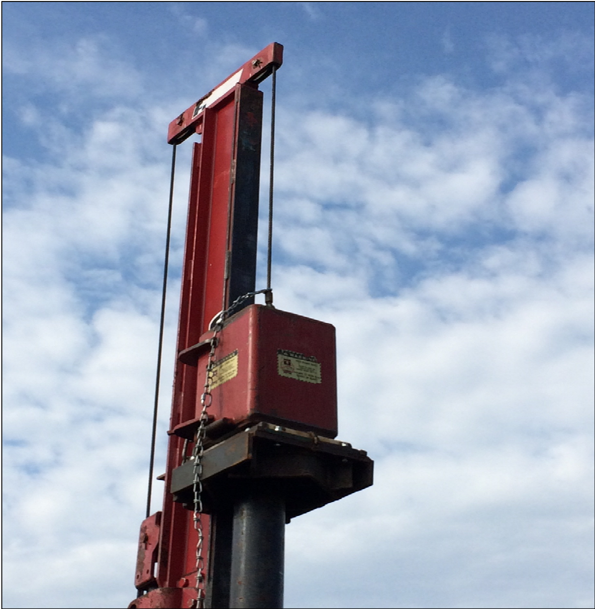
Figure 23. Steel Plate Fabricated to Hold Piles in Place and 500-lbs Hammer.
