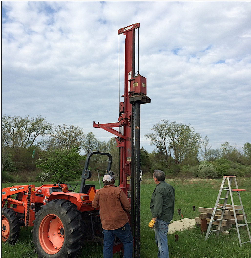
Figure 24. Pipe pile Installation at the HHF Site.
