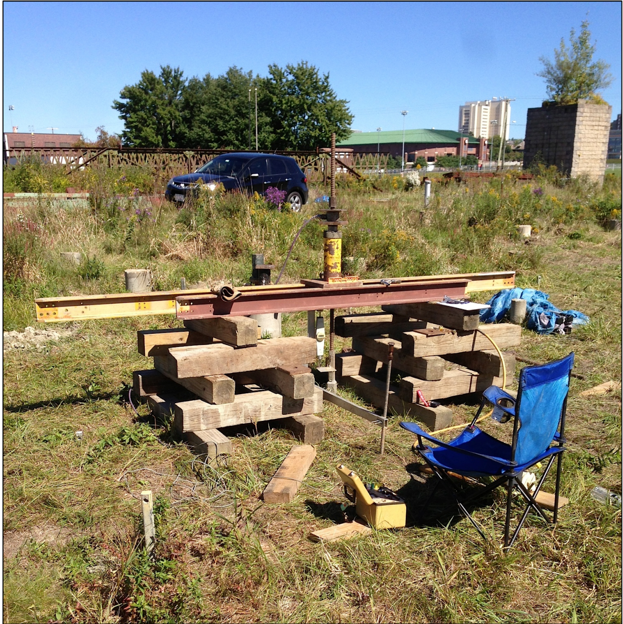
Figure 26. Uplift Load Test Frame Set Up at DOE Site.
