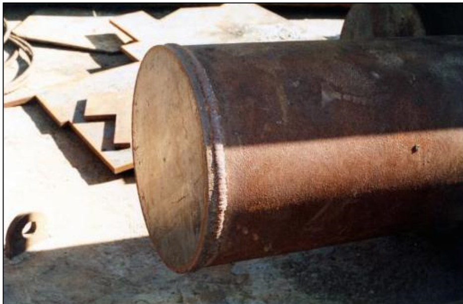
Figure 5. Closed-End Pipe Pile
