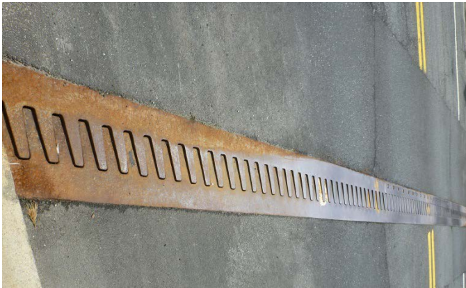
Figure 2.18: Finger Joint Completely Closed at 75°F
