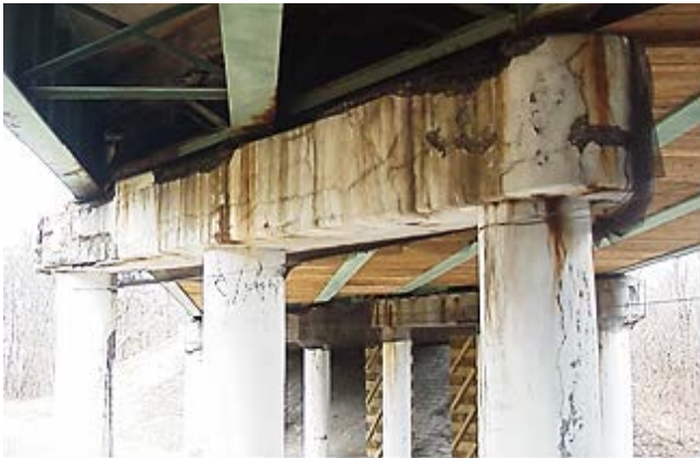
Figure 2.2: Section Loss, Rust Holes and Corrosion Cracks at Deck Joint
