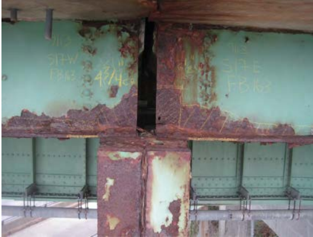
Figure 2.2: Section Loss, Rust Holes and Corrosion Cracks at Deck Joint
