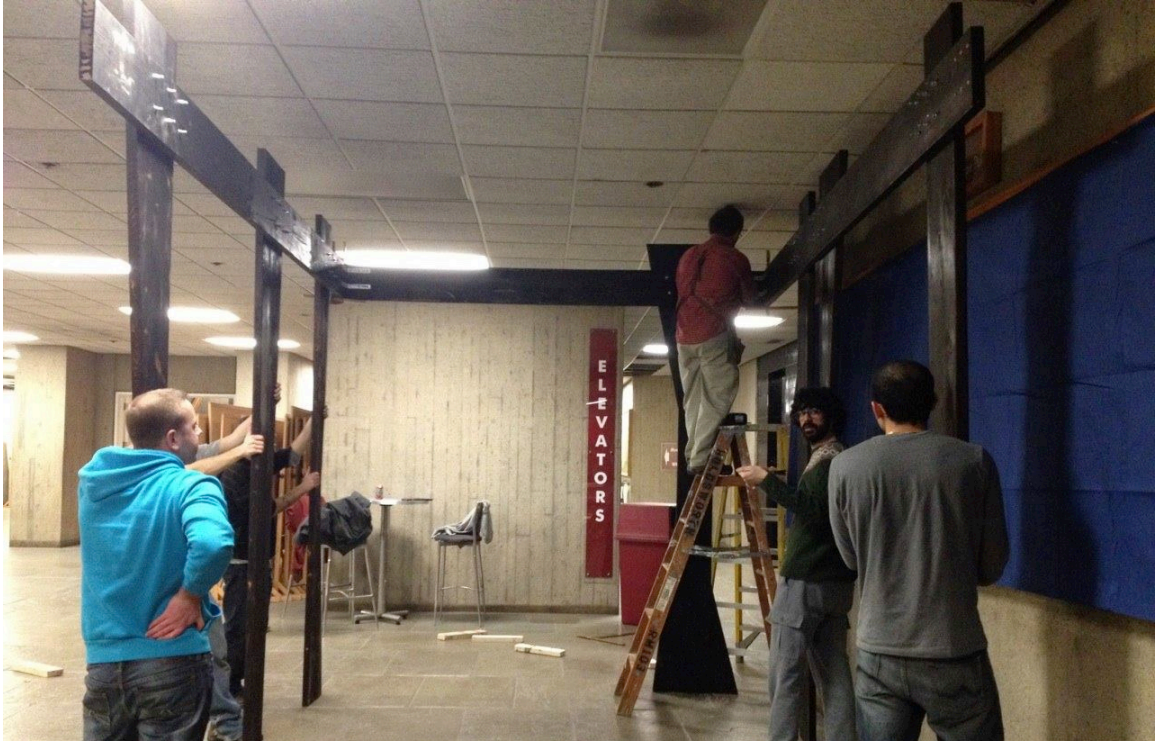
Figure 4.5: The assembly process of structural elements (Image credit by the Author)
