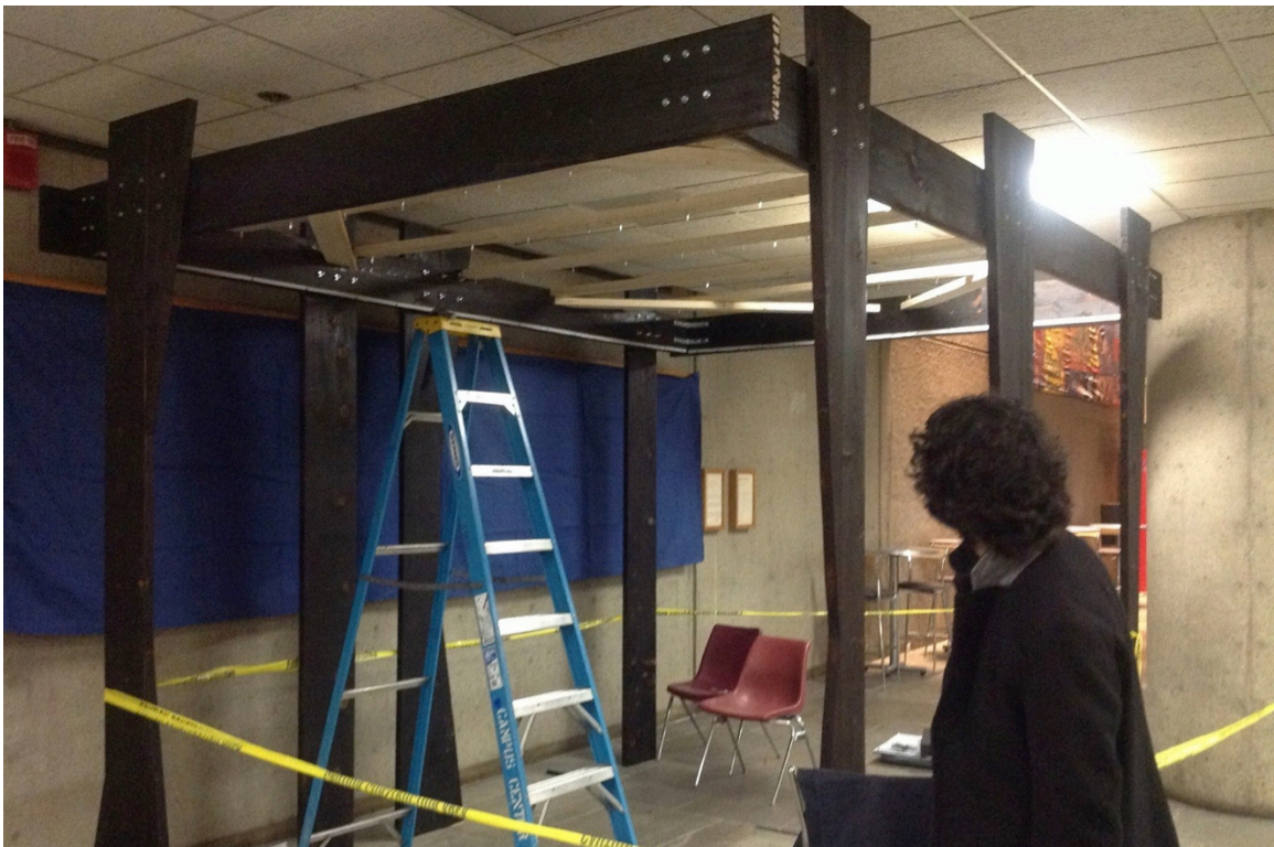
Figure 4.6: The structure of the Intervention; a diagonal connection at corners for creating a rigid connection (Image credit by the Author)
