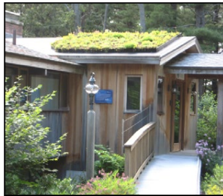
Green roof - one planted with vegetation that absorbs some of the rain that falls on it
