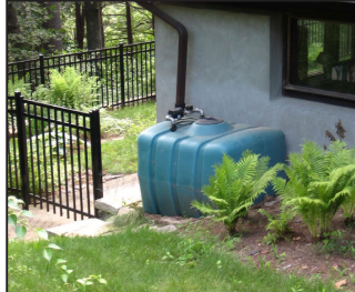
Rain barrel - a container that stores water for later use
