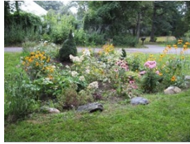
Rain garden — a shallow depression in the ground that collects stormwater, and can be planted with shrubs or flowers
