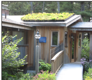
Green roof - one planted with vegetation that absorbs some of the rain that falls on it
