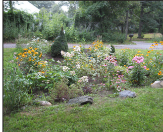
Rain garden - a shallow depression in the ground that collects stormwater, and can be planted with shrubs and flowers
