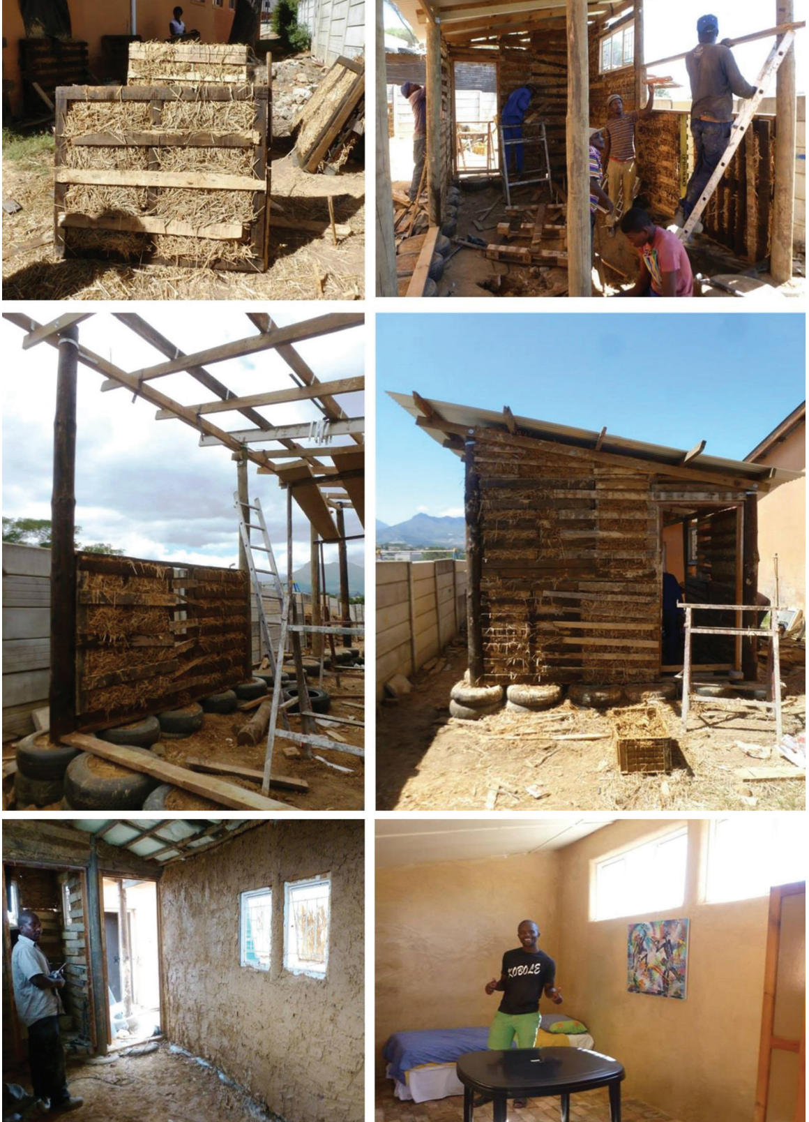
Figure 2: HAPPI ISHACKIV construction (Image credit: HAPPI Organization)
