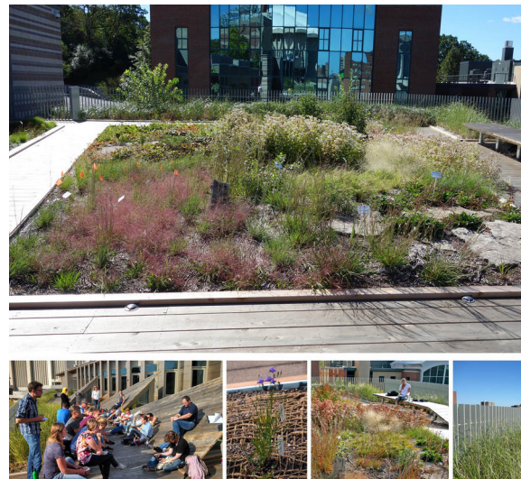
Figure 31: Green Roof of the Gateway Center. Courtesy of AIA.org
