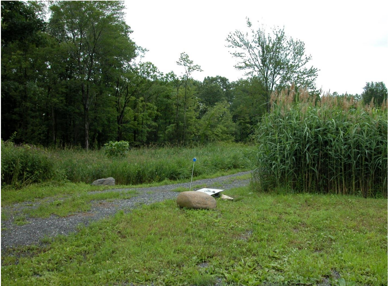
Photo 6 Lloyd Vegetated Sand Beds (Courtesy of NEWS-USA 2006)
