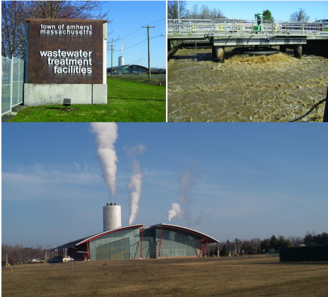
Photo 1, 2, & 3 Amherst Wastewater Treatment Plant (Courtesy of Treatment Plant Operator 2013)
