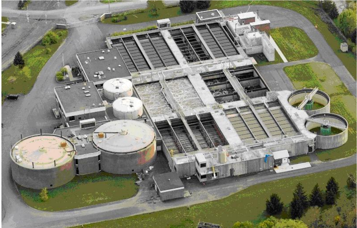
Photo 4 Ithaca Area Wastewater Treatment Facility (Courtesy of the Ithaca Journal 2008)
