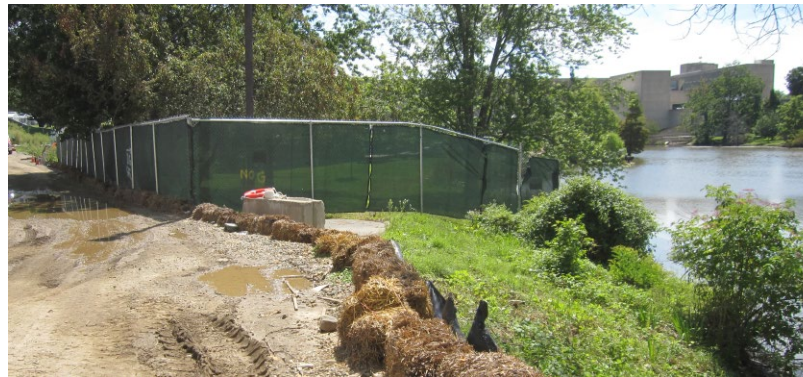
EROSION & SEDIMENTATION CONTROLS PROTECT THE CAMPUS POND FROM CONSTRUCTION RUN-OFF
