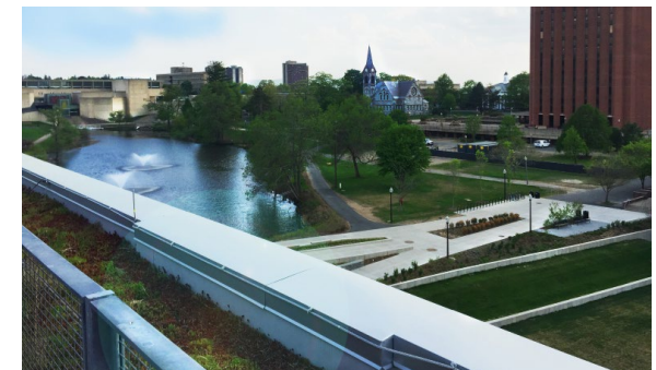
LIGHT COLORED WALKWAYS HAVE A LOW SRI. PHOTO TAKEN FROM ILC ROOFTOP
