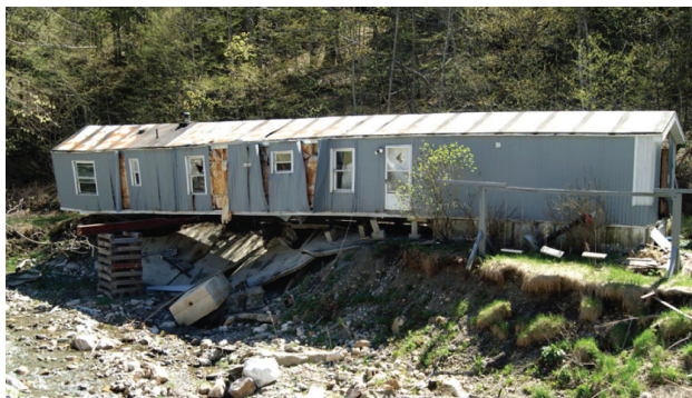
Crumbling house on Flower Brook, near the confluence of the Mettowee River, in Pawlet, Vermont after Tropical Storm Irene, 2011
