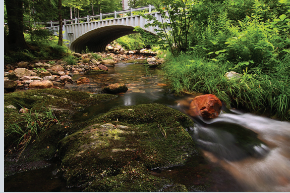
This new crossing was installed in 2008 on Bronson Brook through a partnership of federal, state and non-profit agencies. It cost less than an in-kind replacement. During Irene, large wood and boulders passed beneath this fish-and-wildlife-passage-friendly structure without damaging it.
