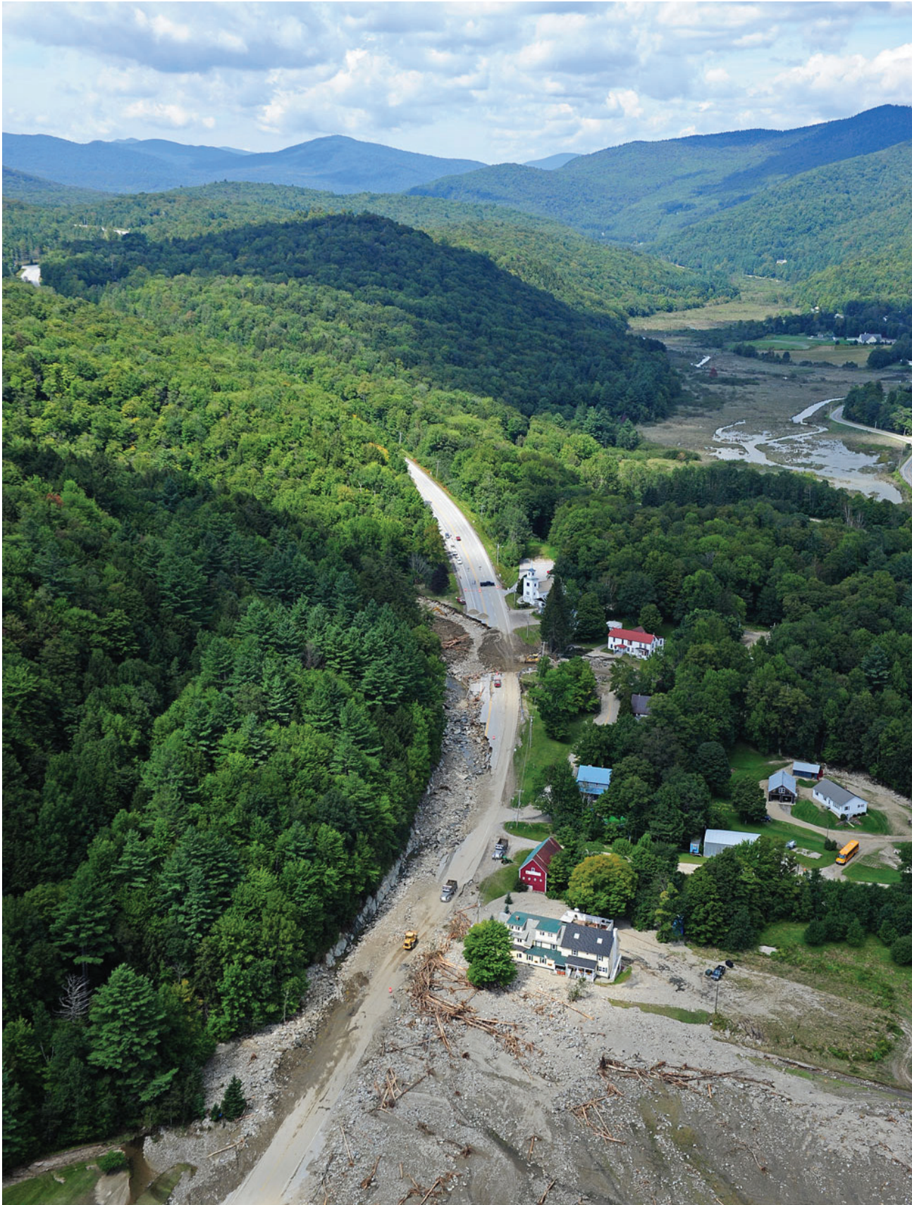
US Route 4 in Vermont was no match for the force of water, sediment and debris raging down into and along the Ottaquechee River during Tropical Storm Irene.
