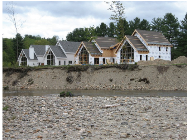
Houses at high risk of fluvial hazards, under construction over an eroding bank in Stowe, Vermont.
