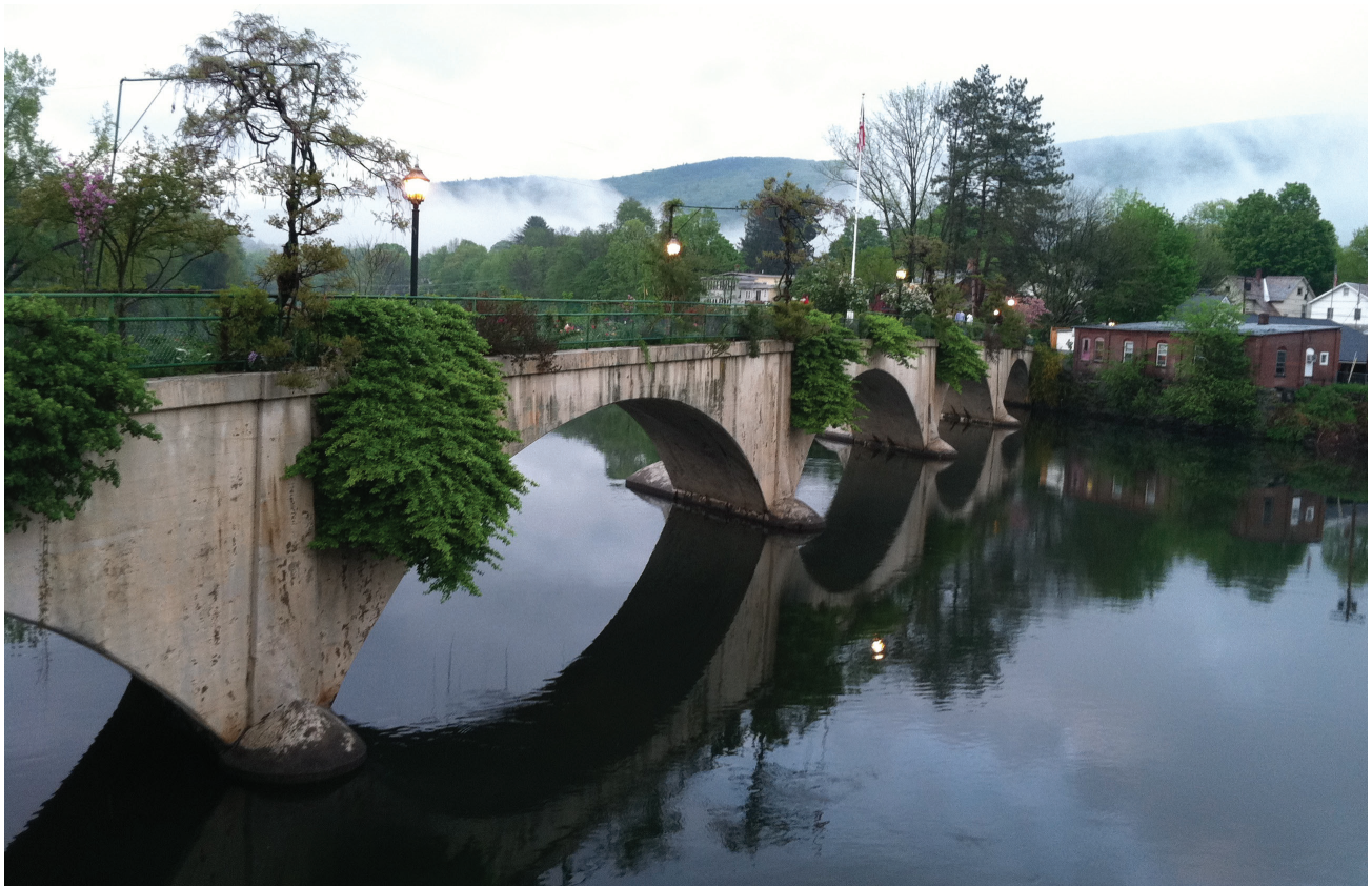
The Bridge of Flowers in Shelburne Falls, Mass. This photo highlights just one of the many riverside landscapes that define New England communities. In contrast to the serenity shown in this picture, during Tropical Storm Irene in August 2011, the raging Deerfield River nearly filled the bridge's arches. Because the bridge was built well to pass water, sediment and debris, it remained whole, but the torrent caused significant damage to riverside properties. By helping New England communities to become river-smart, we can ensure that when our beloved rivers flood, more of our homes, buildings and infrastructure remain resilient, and the region's rivers support rather than ravage the iconic places and landscapes that we love in New England.
