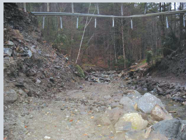
Townshend road crossing. The left-hand photo shows the crossing after Tropical Storm Irene. A wire with dangling posts – the remains of a guard rail – was all that was left of the road. The former crossing had an oval pipe ("plate arch") culvert which failed catastrophically. The new crossing, built to Vermont's 2010 standards, is on the right.
