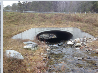
Townshend road crossing. The left-hand photo shows the crossing after Tropical Storm Irene. A wire with dangling posts – the remains of a guard rail – was all that was left of the road. The former crossing had an oval pipe ("plate arch") culvert which failed catastrophically. The new crossing, built to Vermont's 2010 standards, is on the right.
