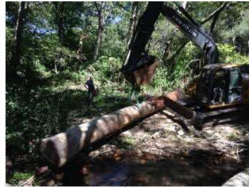
30k lb excavator placing log in stream at 3500
