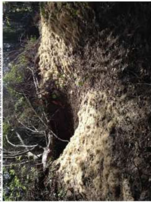
PP12 facing east at ag drain culvert and levee berm on 3/25/2013
