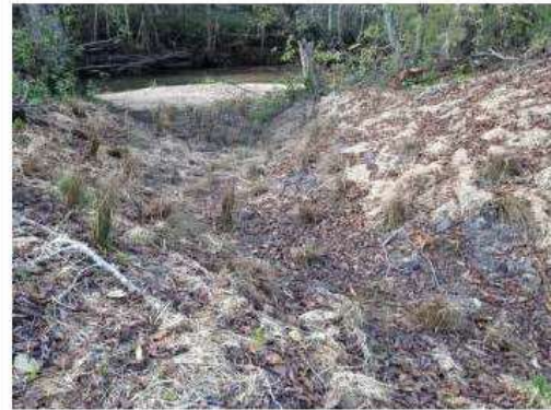
Looking west at alcove feature at 4250.
