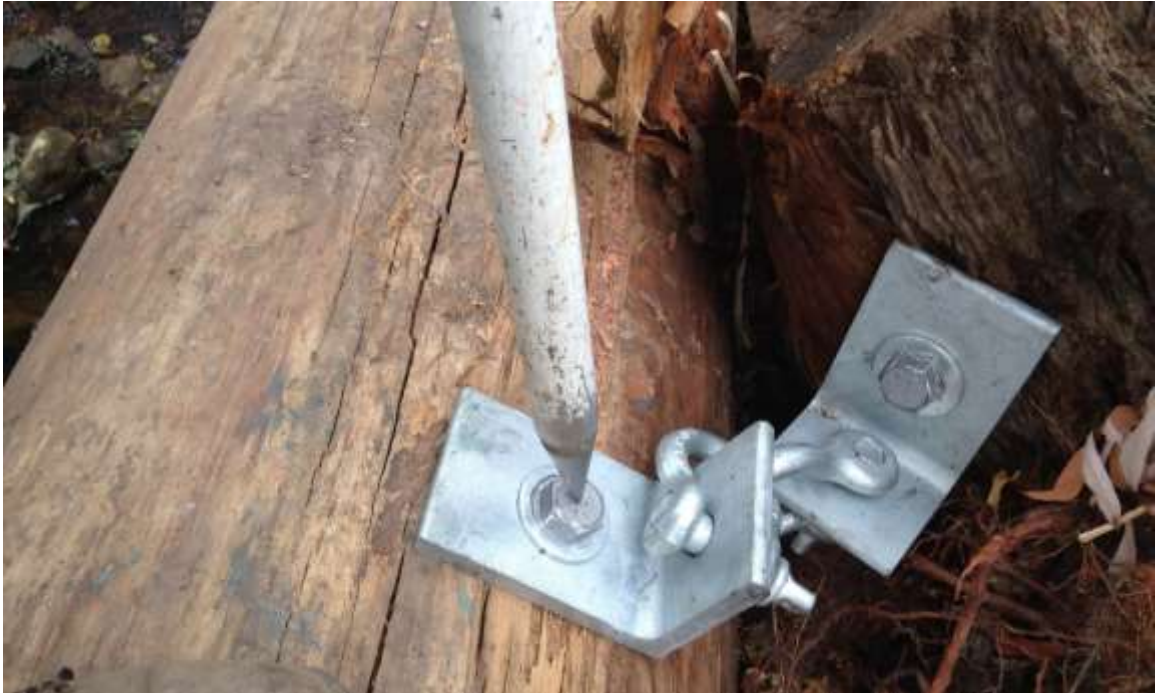
Figure 17. Surveying bolt heads.
