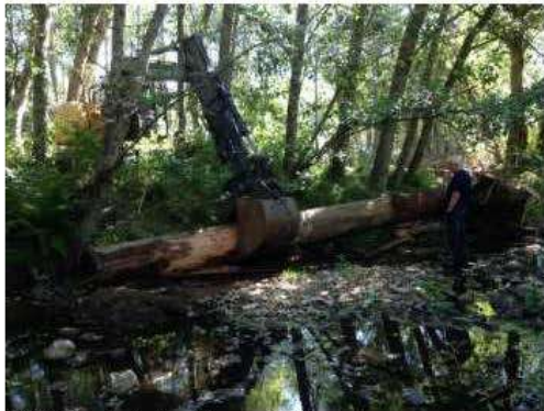
30,000 lb ex placing log in stream at 380
