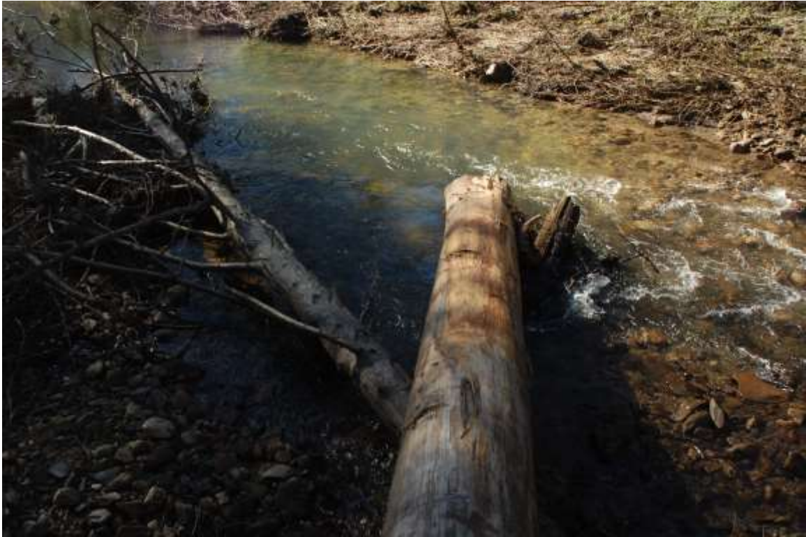
Figure 22. Photo of LWC at 2750 following stormflow showing deposition of cobbles, pool scour, and debris racking.
