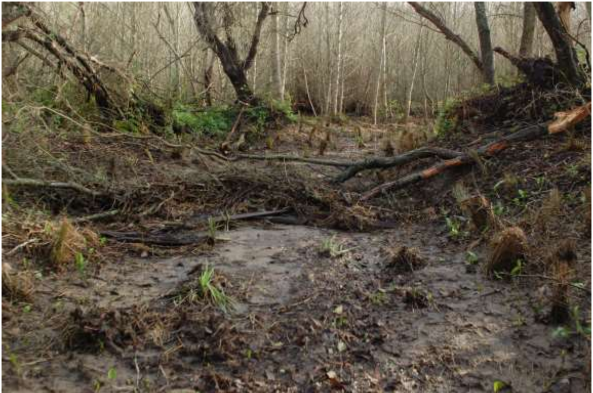
Figure 24. Looking east at debris racked across the throat of the breach at 2000 on 12/18/2014. Scotts Creek is directly behind the vantage point.
