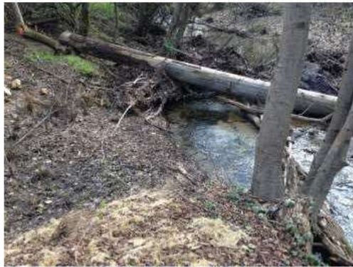
PP2. Looking south at alcove and LWC (3300)
