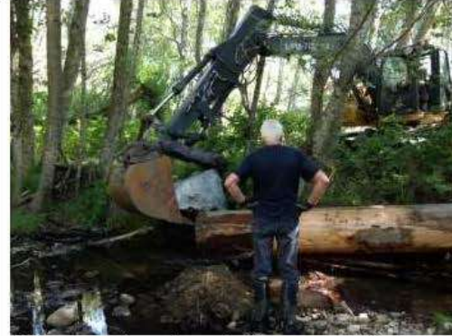
30k lb excavator placing three ton boulder in stream at 3800
