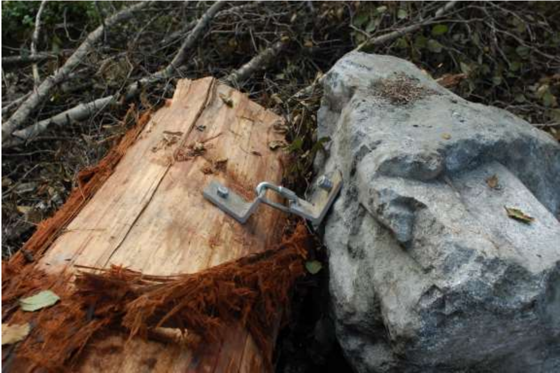
Figure 12. Log-boulder coupler.
