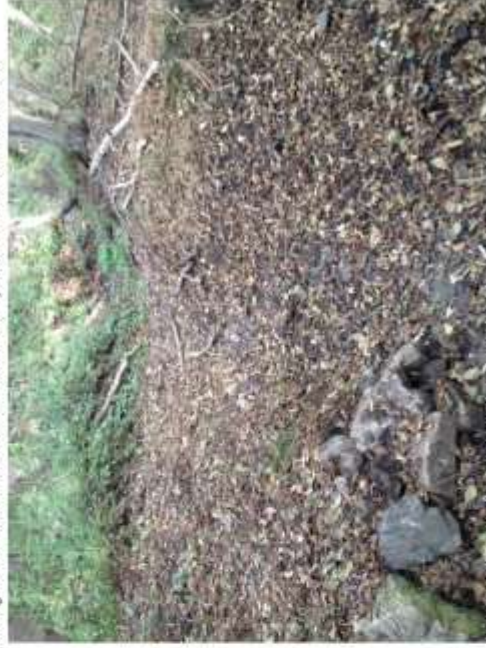
Close-up photo of rock armoring on 9/30/14, facing northwest. Rock was unearthed during excavation and reused. No rock was imported to construct this feature.
