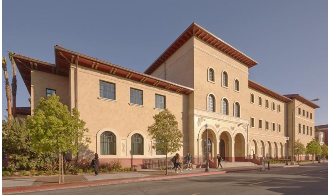
Figure 16: USC Cinematic Arts Project 40
