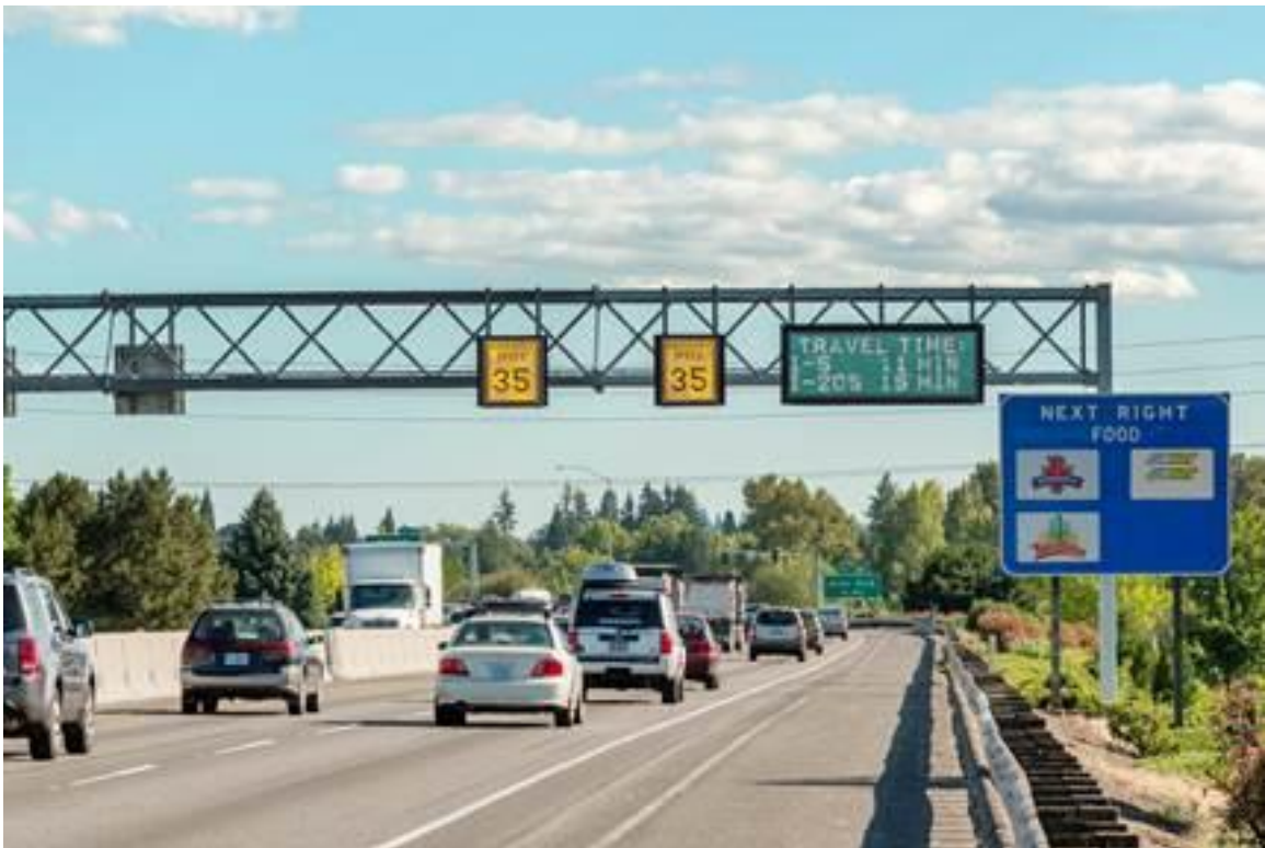
Figure 16: OR 217 VSL Signs on Sign Gantry
