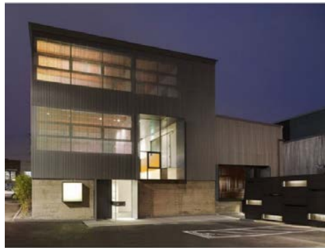
Figure 6.3: 355 11 th Street Perforation (ArchDaily, 2015)
