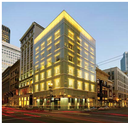
Figure 2.12: 185 Post at Night (Architecture Record, 2015)
