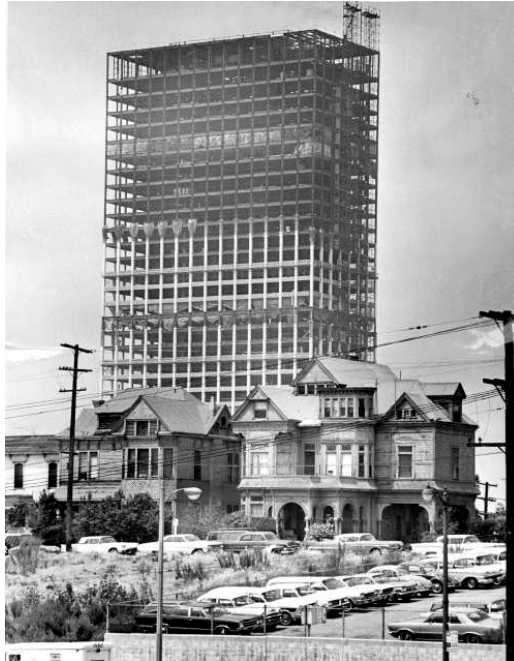
Figure 3.4: Union Bank Plaza during Construction (Los Angeles Times, 2015)
