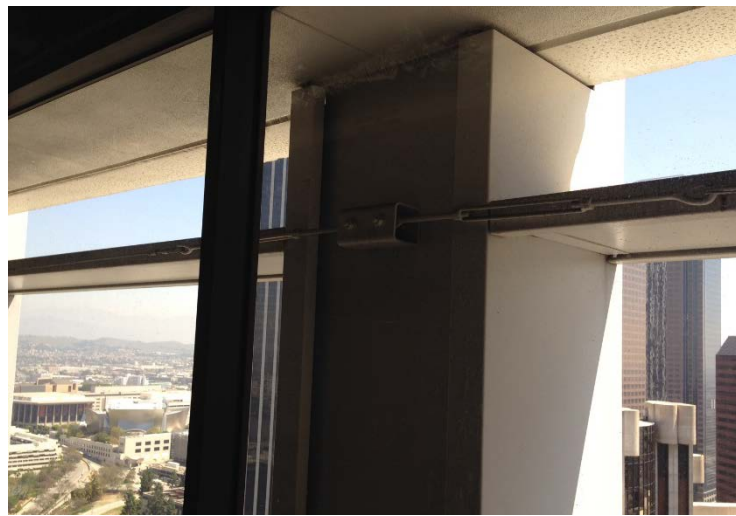
Figure 3.8: Union Bank Plaza - Safety Cable Tie-off (Heneghan, 2014)
