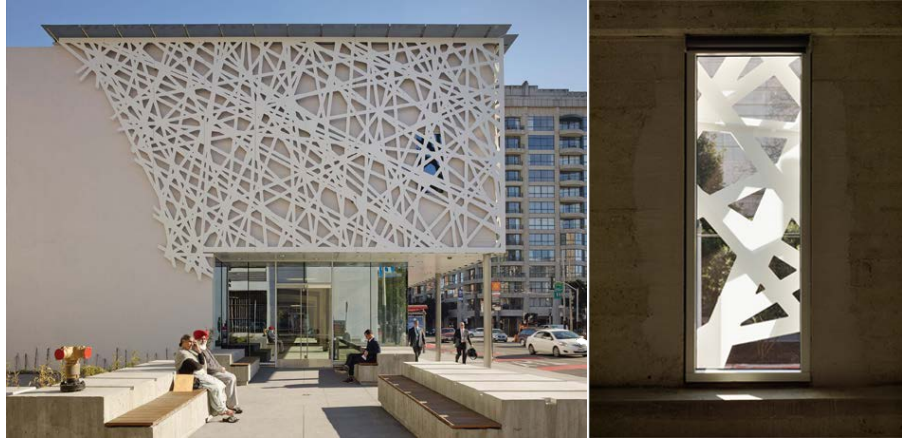
Figure 2.8: 690 Folsom Street Screen Wall Window Feature (Bloszies, 2015)
