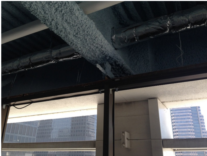
Figure 3.7: Union Bank Plaza - Glazing Termination Detail (Heneghan, 2014)
