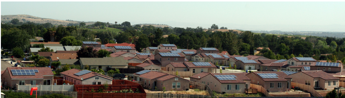
Figure 1. People's Self Help Housing Development in Templeton, CA powers up with the Solar Affordable Housing Program during GRID Alternatives' Central Coast's first Solarthon in 2011. Source, Author.
