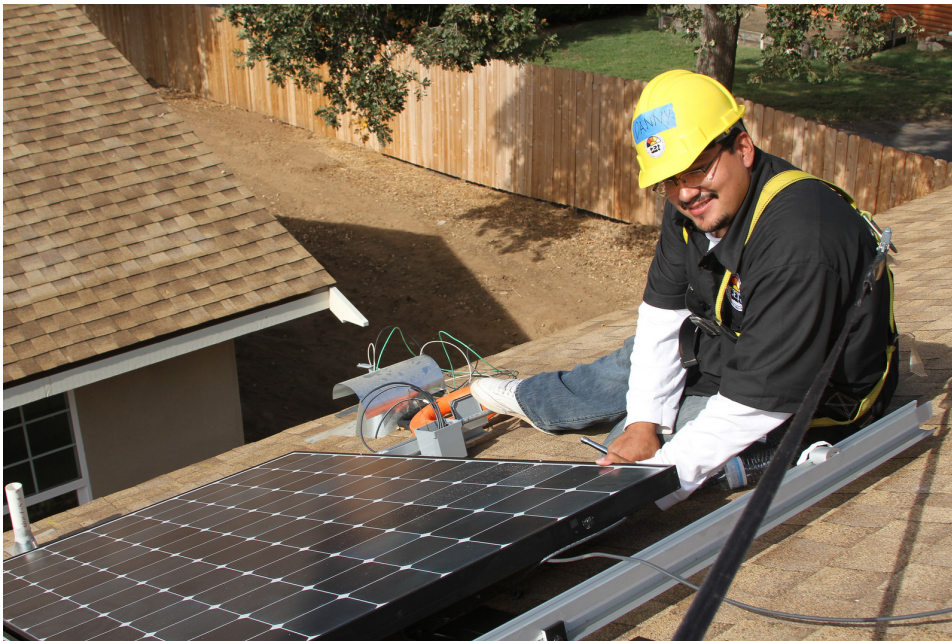
Figure 2. Danny, a job trainee from Center for Employment Training installs solar electric panels in Atascadero, CA, (GRID, 2014).
