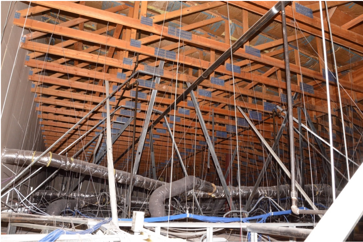
Figure 7: Second floor attic, north side of the building, looking west
