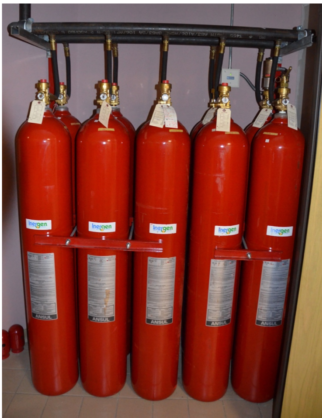
Figure 31: Inergen cylinders and clean agent spray nozzle
