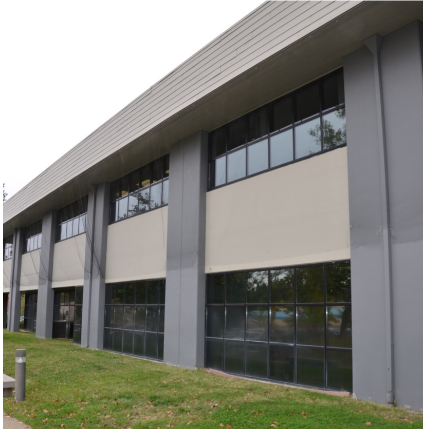
Figure 5: South exterior wall, west side of the building
