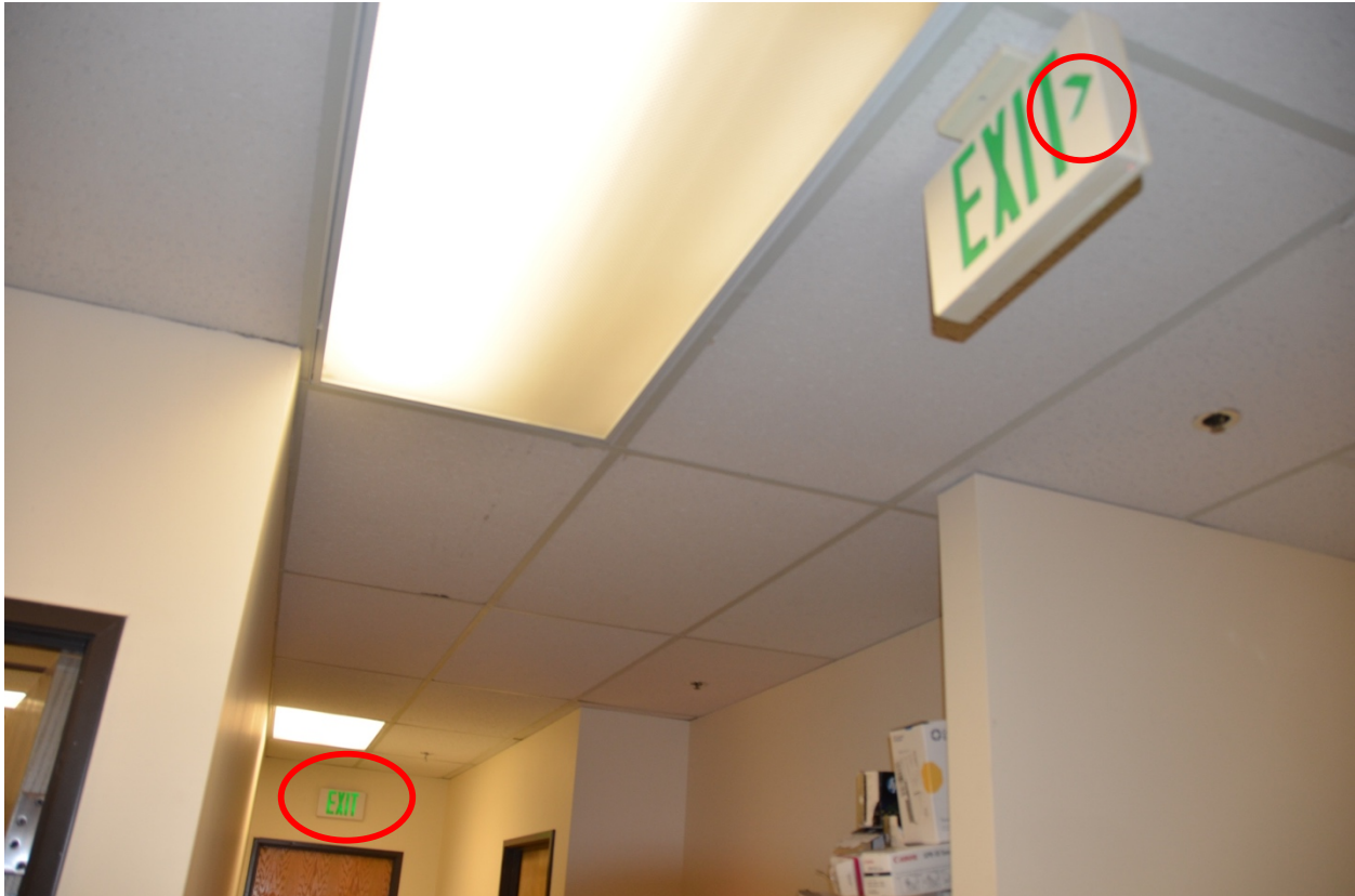
Figure 12: The exit sign's directional arrow in the CDA pointing away from the nearest exit
