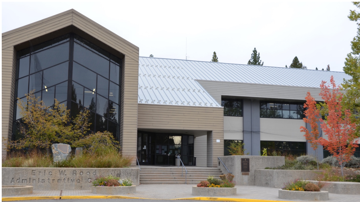
Figure 6: South portion of the roof at the front of the building
