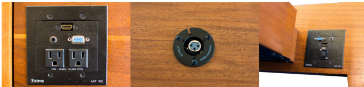
Figure 77. AV connectivity at the top of lectern (left and middle) and at the base (right)
