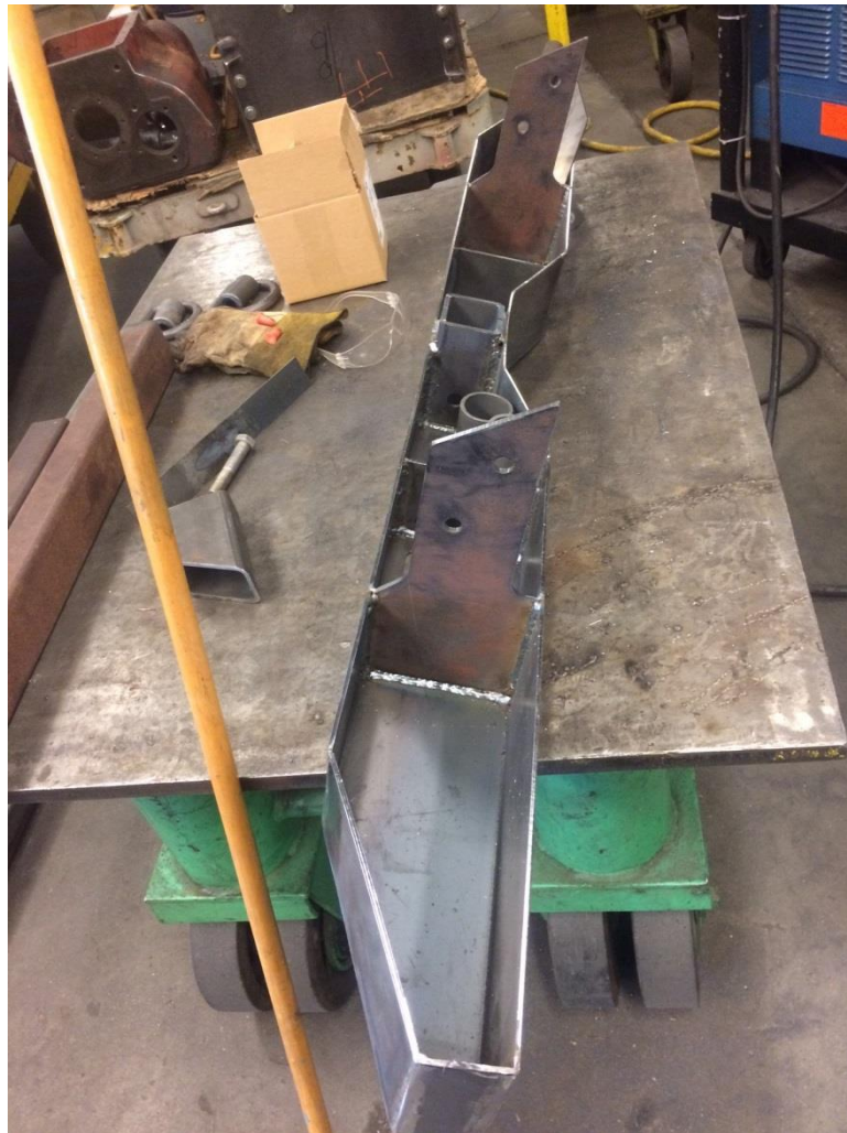
Figure 26. Bumper channel with side flanges, mounting plates and channel flanges welded in place.
