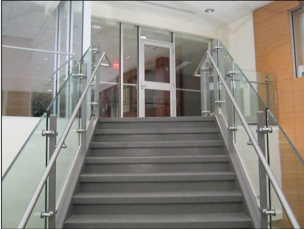
Figure 15: Atrium stair showing separation between the atrium and third floor office space
