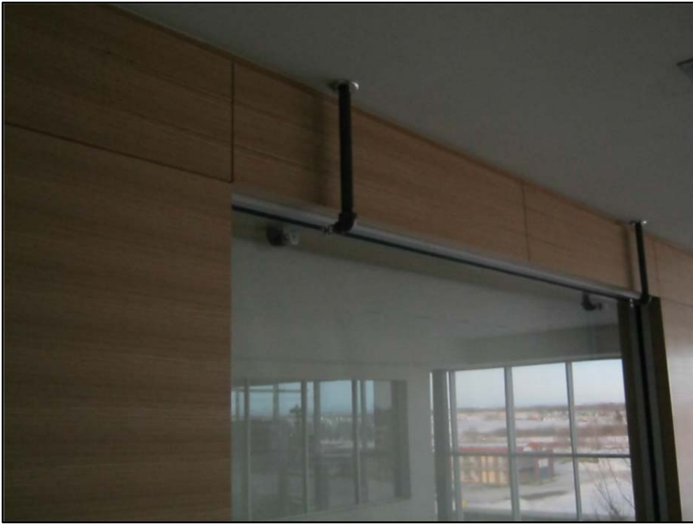
Figure 18: Gazing protection in the atrium space
