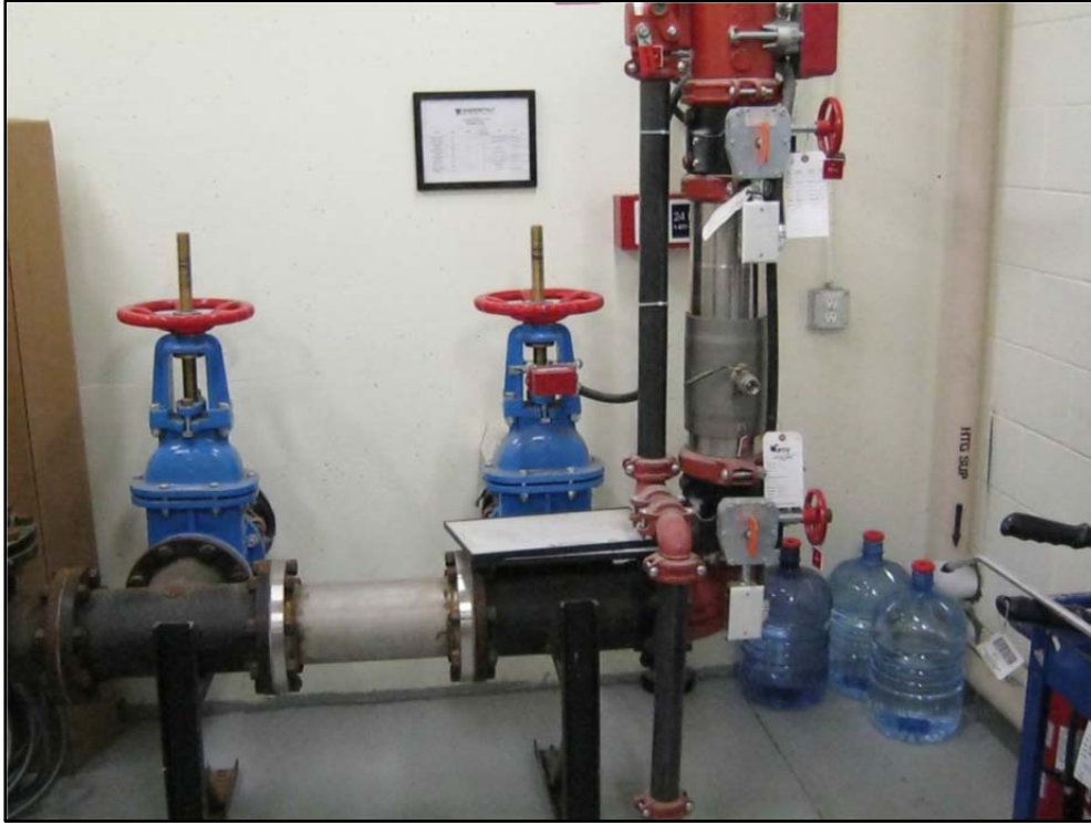
Figure 25: Main water supply arrangement
