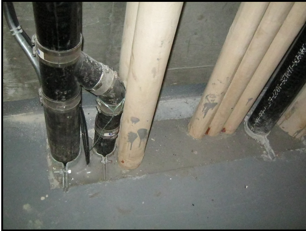
Figure 45: Typical floor penetration
