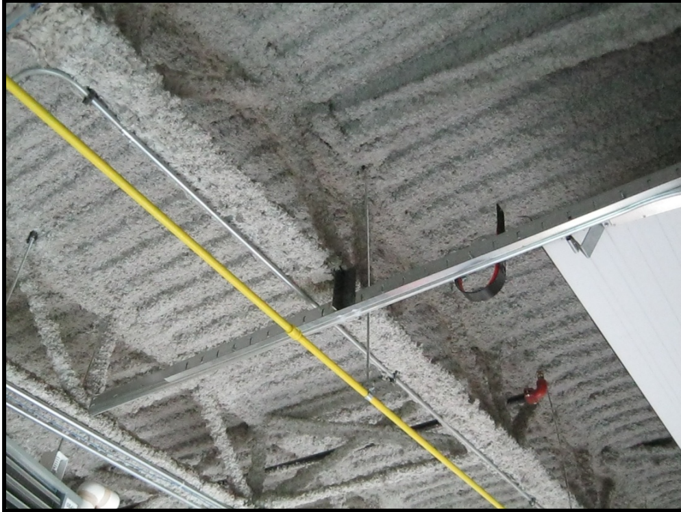
Figure 38: Fire proofing on joists and the underside of the floor assemblies
