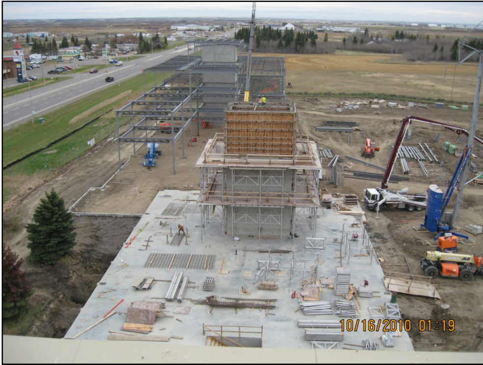
Figure 10: East and west exit enclosures during the project building construction.
