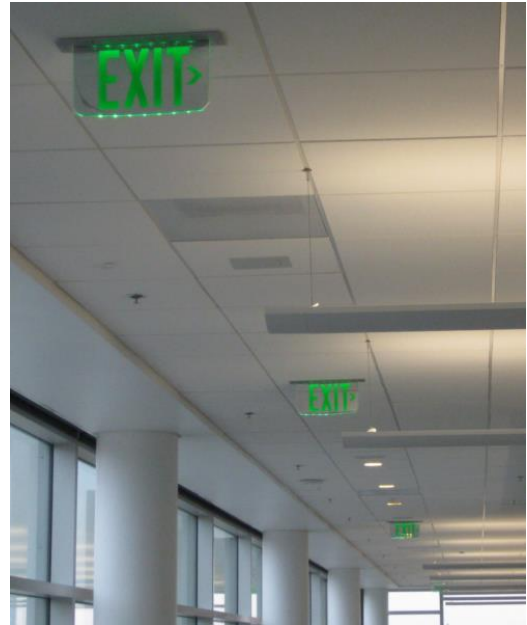
Figure 13: Photo of Existing Exit Signs
