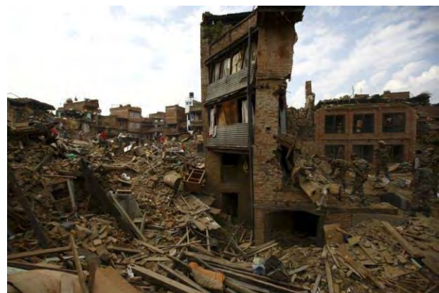
Figure 4: Adobe building after the earthquake
