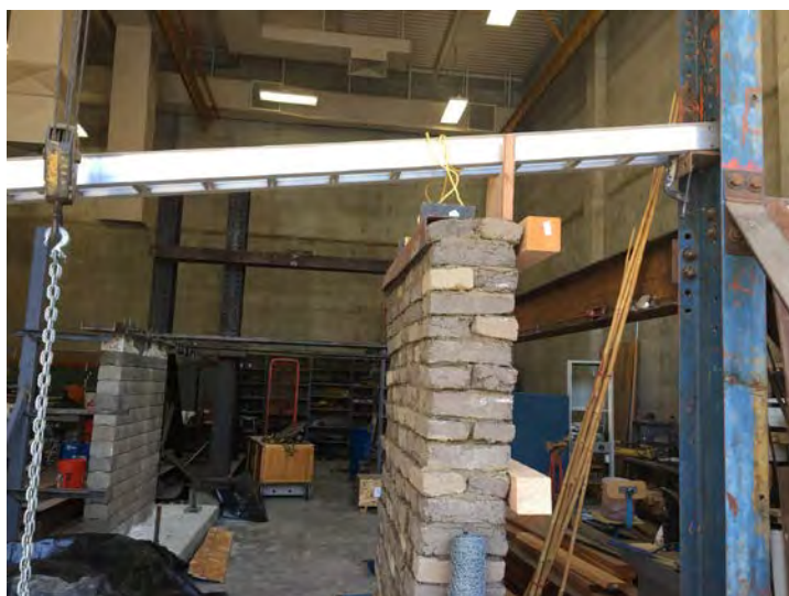
Figure 28: Adobe wall test set-up – Side View
