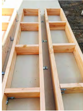
Figure 20: Adobe brick formwork
