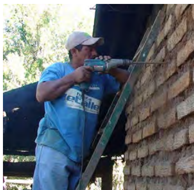
Figure 11: Drilling into Adobe wall
