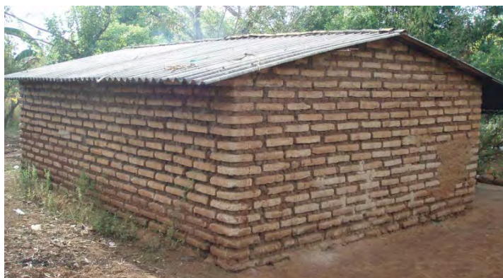
Figure 12: Adobe wall in Peru – Pre-Retrofit
