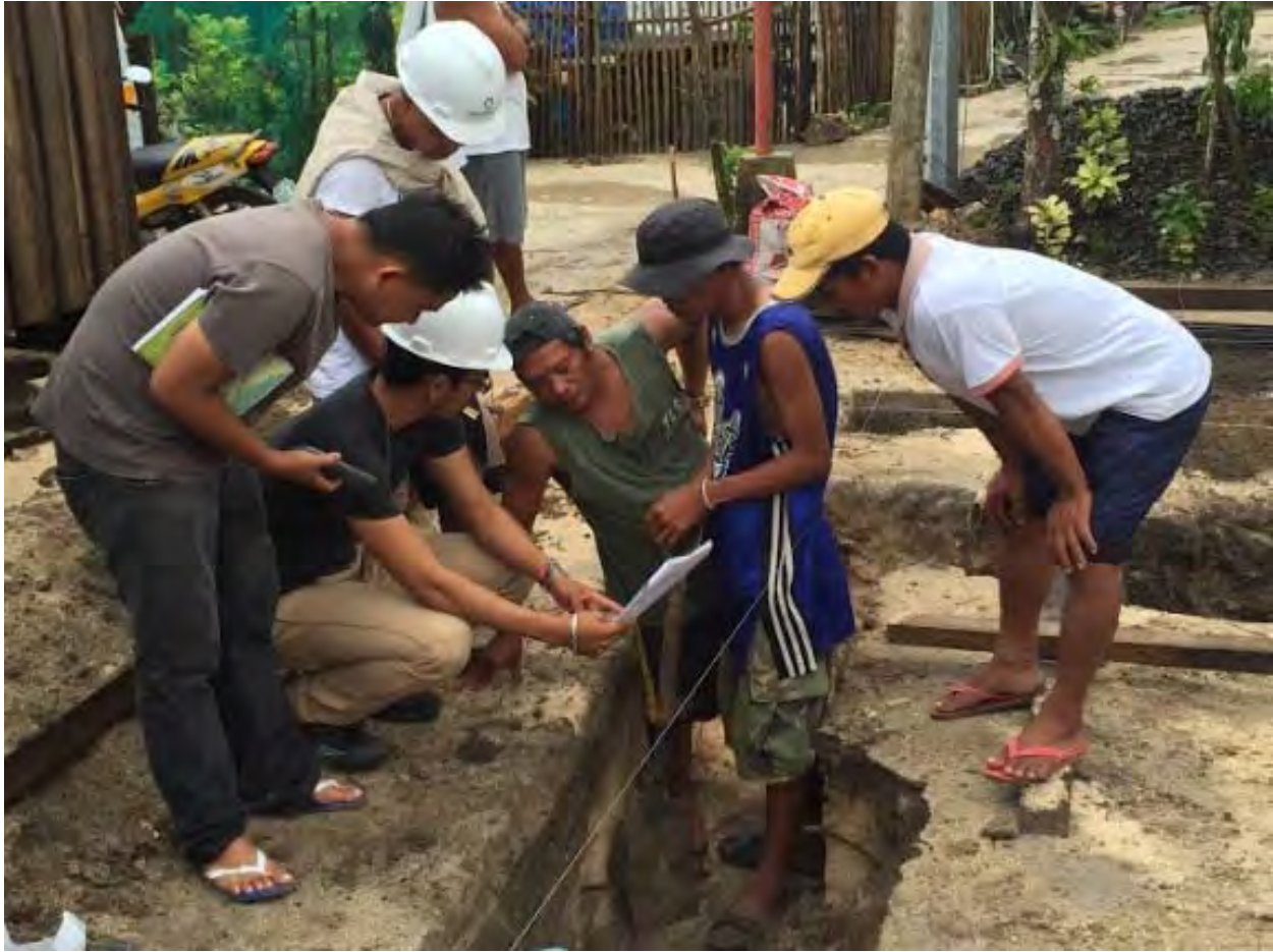
Figure 16: This image reveals the eagerness in learning as Gilbert Appa, The Build Change Resident Engineer, explains the structural details of the foundation to the locals.
