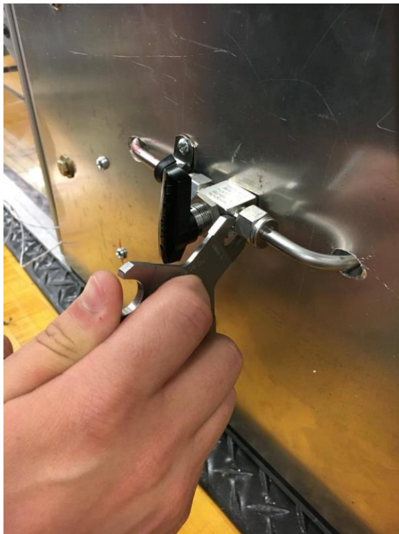
FIGURE 29. CHECKING SWAGELOK FITTING WITH NO-GO GAUGE
