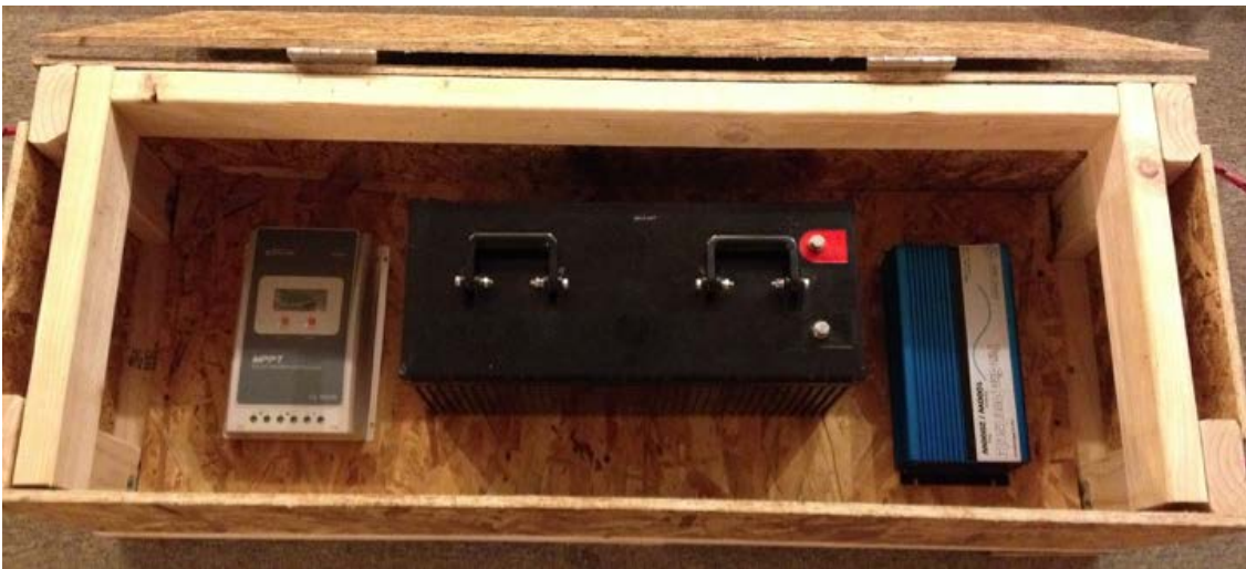
Figure 4.16: Completed Housing for Electrical Components
