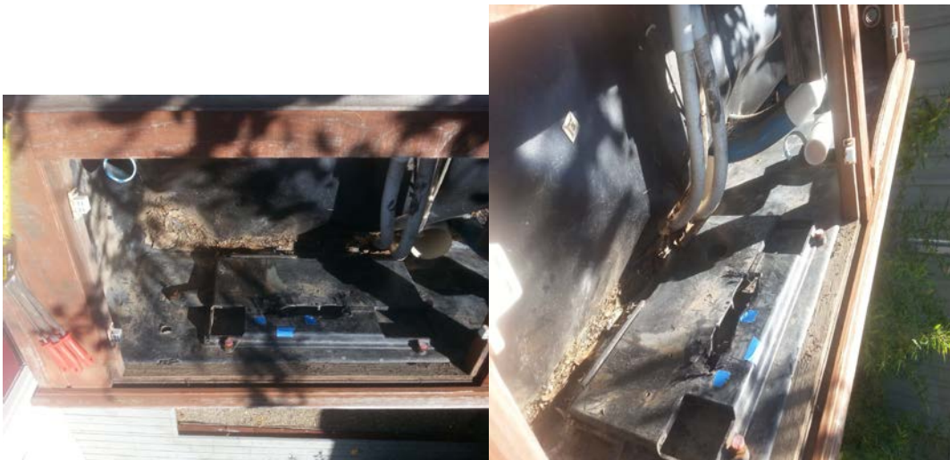
Figure 4.1: Hot Tub with Pump and Wiring Removed
