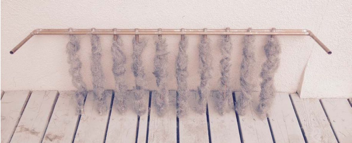
Figure 4.14: Prepped Copper Tubing
