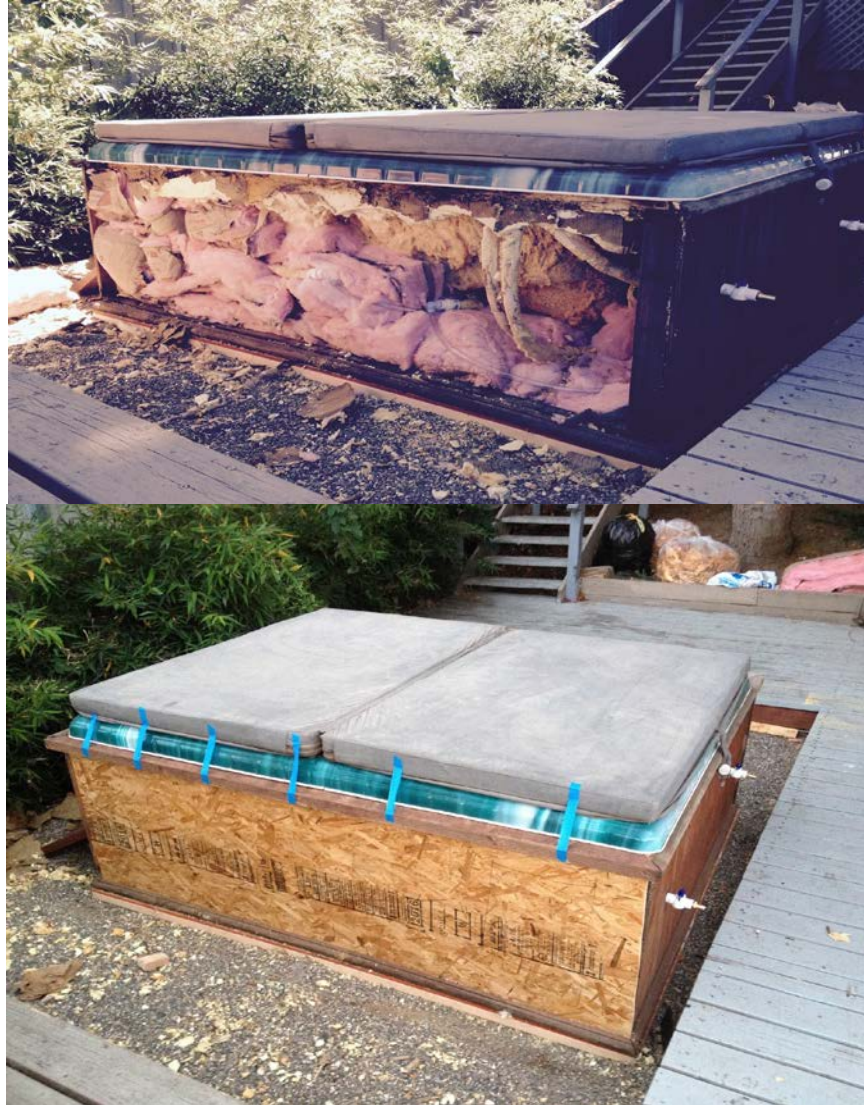
Figure 4.9: Pre and Post Finished Side Panel
