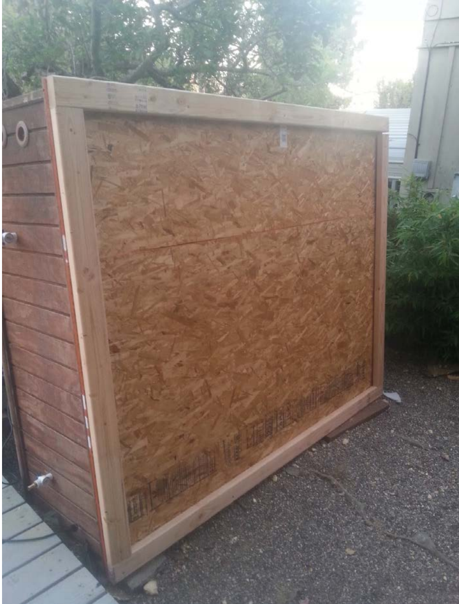
Figure 4.8: Finished Hot Tub Base
