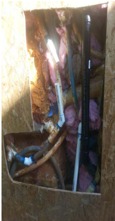
Figure 4.7: Hot Tub Plumbing Leak Repairs
