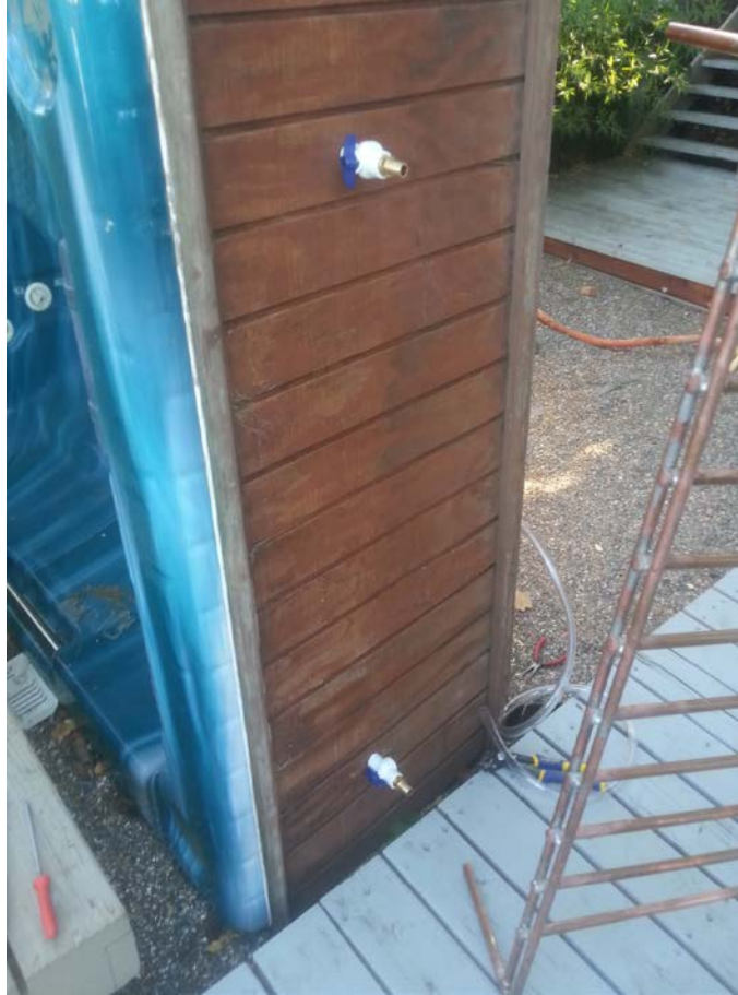
Figure 4.6: Final Plumbing for Hot Water Heater Assembly
