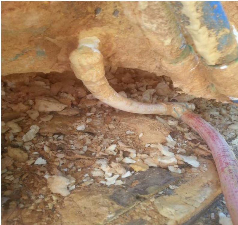
Figure 4.5: Existing Port chosen for Hot Water Heater Assembly
