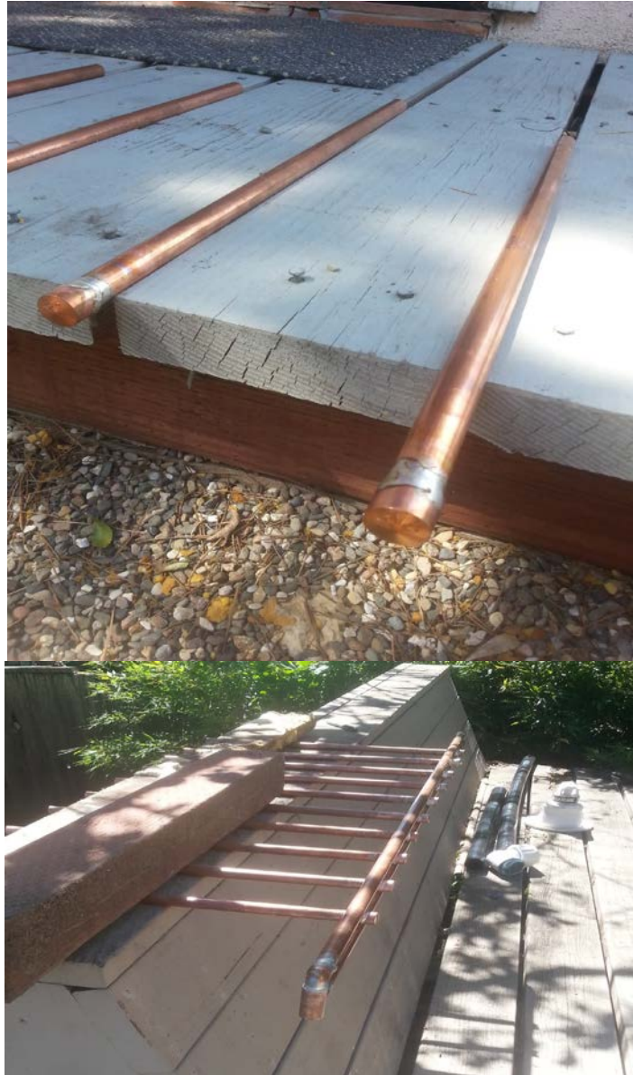
Figure 4.12: Heat Exchanger Construction
