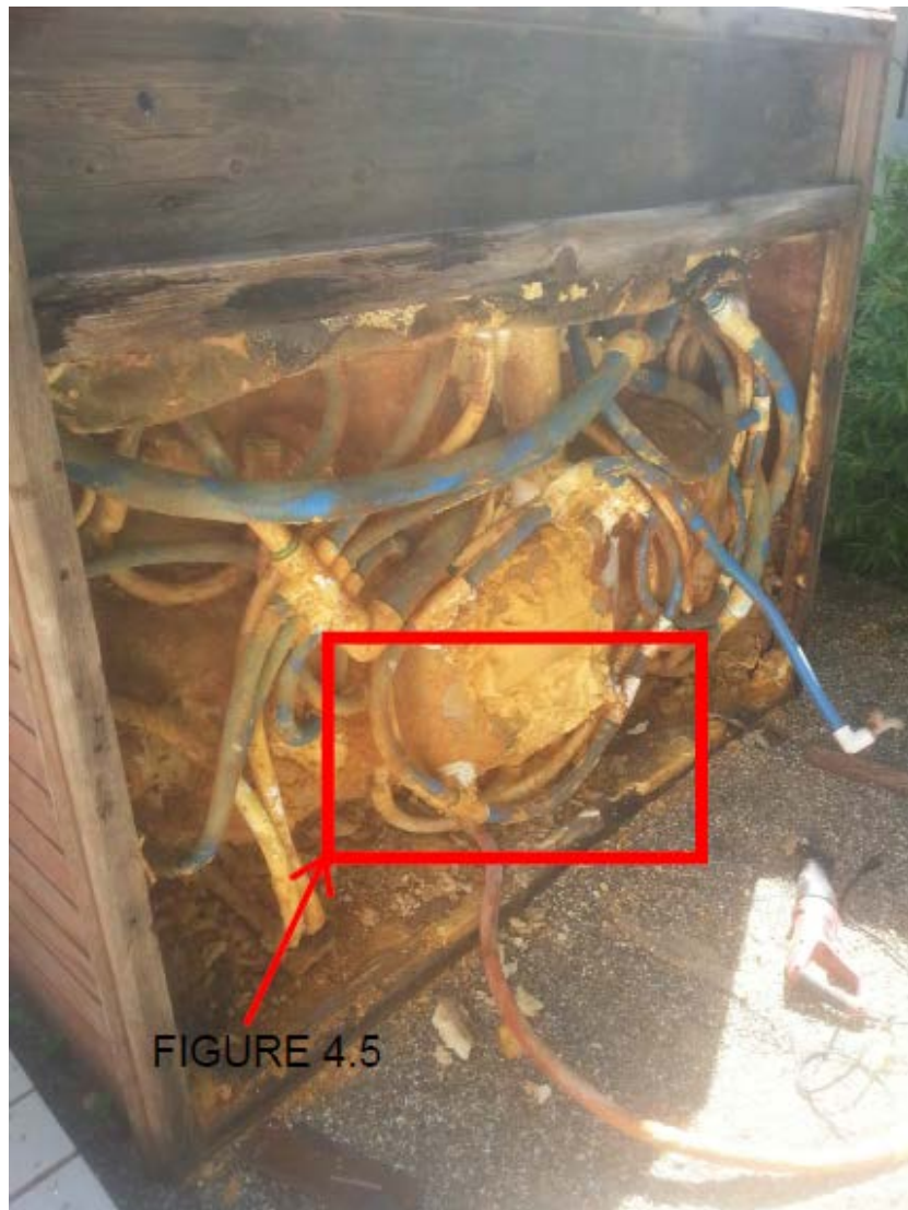
Figure 4.4: Existing Hot Tub Plumbing (Insulation Removed)
